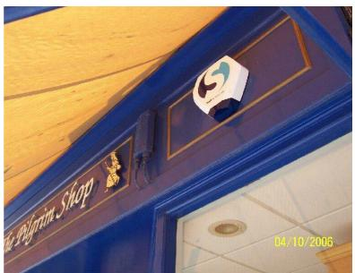
The left hand illustration shows how the cell is concealed behind the awning of the shop. The right hand illustration shows the cell behind the awning, to the right of the shop name and to the left of the burglar alarm, which is larger than the cell.
