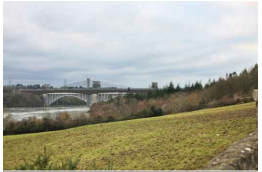
PONT ECSTRADOS DAU LED EXTRADOS TWO-SPAN BRIDGE
