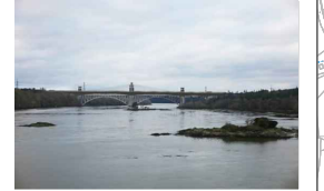
PONT ECSTRADOS DAU LED EXTRADOS TWO-SPAN BRIDGE
