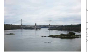
PONT GEBLAU CABLE-STAYED BRIDGE
