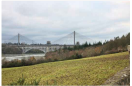
PONT GEBLAU CABLE-STAYED BRIDGE
