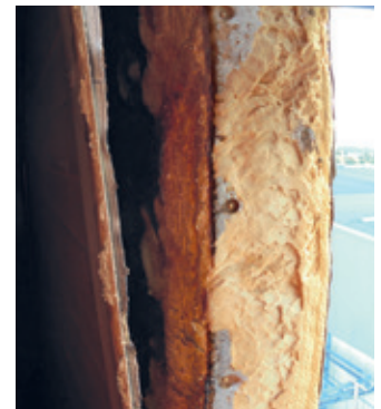
Window removed by Fire Service to ventilate the building to gain access – no fire penetration of core material.
