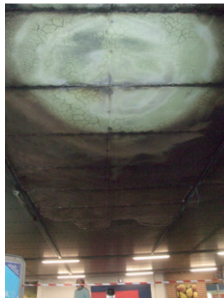
Evidence of direct flame impingement on soffit lining directly above the car.
