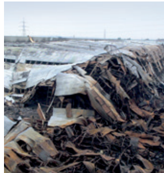
Collapsed south end of building.
