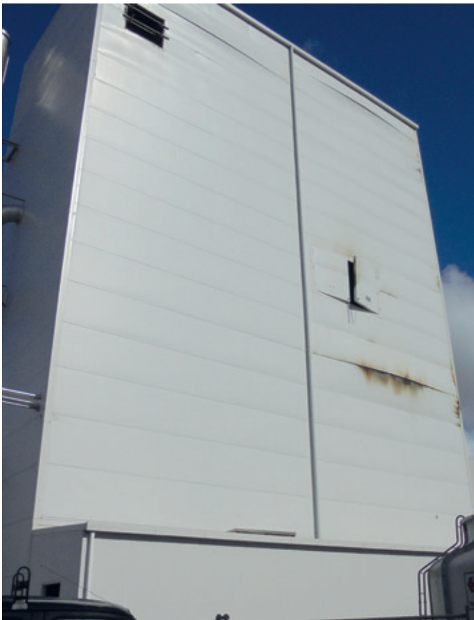
Milk powder drying tower showing external fire damage to panels explosion doors opened manually after fire).
