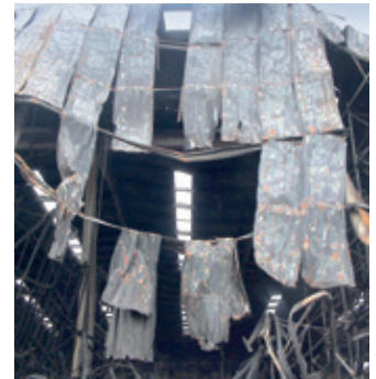
Roof sheeting hanging from severely deformed steelwork.
