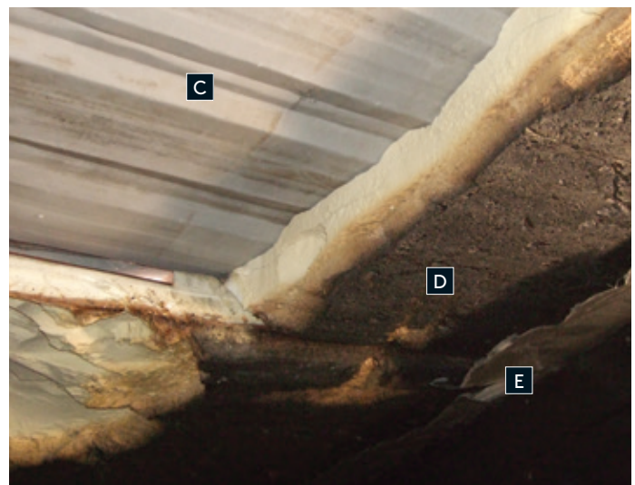
C: Temporary roof covering over hole in roof. D: PIR core showing delaminated lower surface and extent of through-thickness charring. E: Cut edge of lower steel skin of sandwich panel.
