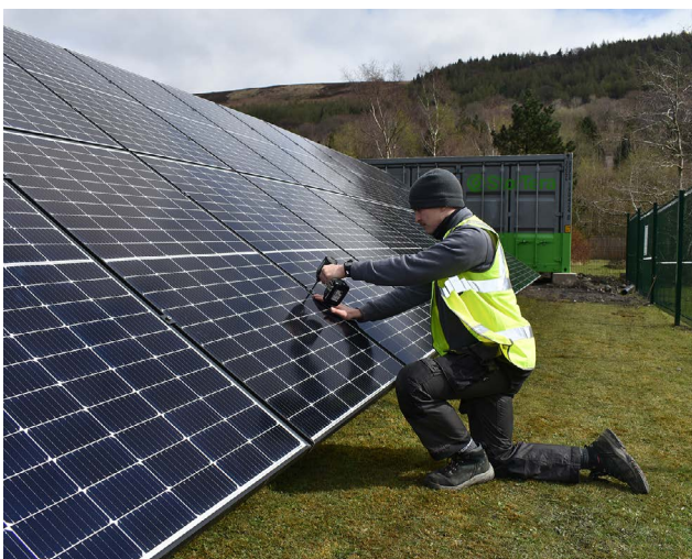
Gosod paneli solar ar safle Parc Busnes Roseheyworth.
