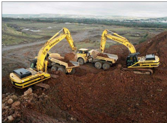
Gweithrediadau Cloddio Tir Earthwork Operations
