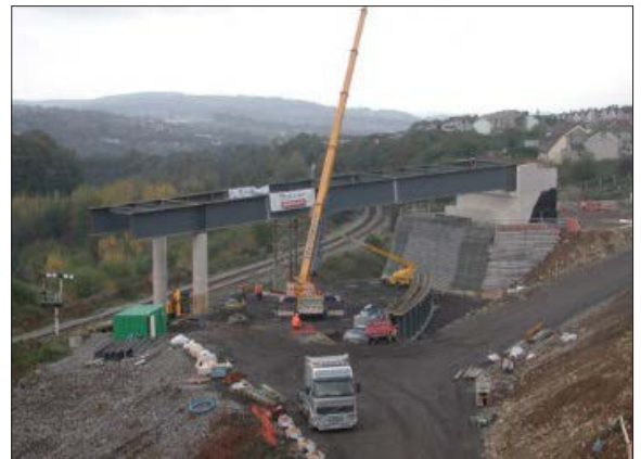
Adeiladu Pont dros Reilffordd Construction of a Bridge over a Railway
