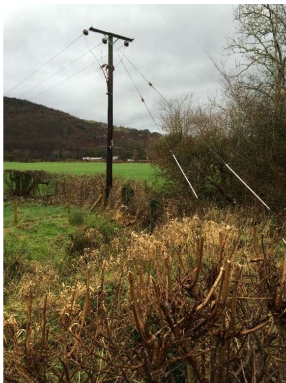
Photo 2 b – Southern drainage ditch looking north east
