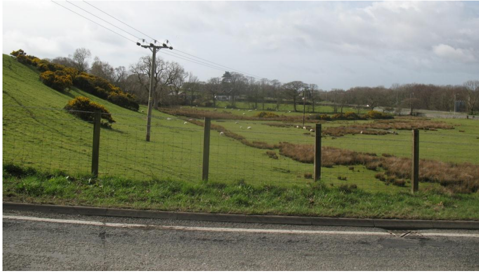
Photo 3: Looking south west from roundabout near Plas Menai at the northernmost extents of the alignment. Section of cutting runs to south east from this locality.
