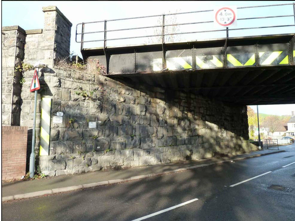
RAILWAY BRIDGE ABUTMENTS: DRESSED MASONRY BLOCKS, UNCOURSED
