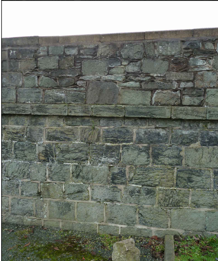
CAR PARK RETAINING WALL: DRESSED MASONRY BLOCKS, COURSED AND UNCOURSED
