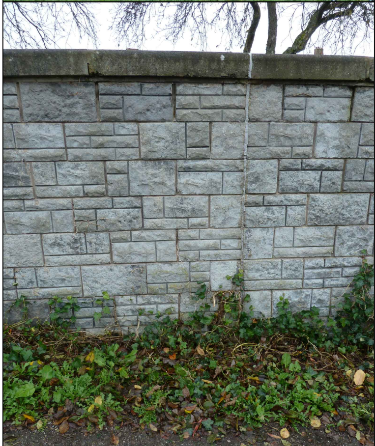
MODERN RIVER BRIDGE ABUTMENTS: CONCRETE FACING BLOCKS, UNCOURSED
