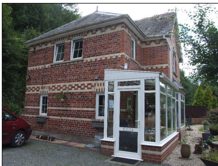
Photo 1 – exterior of the property, view from the north-west
