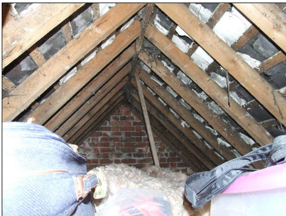
Photo 3 – View of inside the loft
