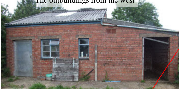
The outbuildings from the west
