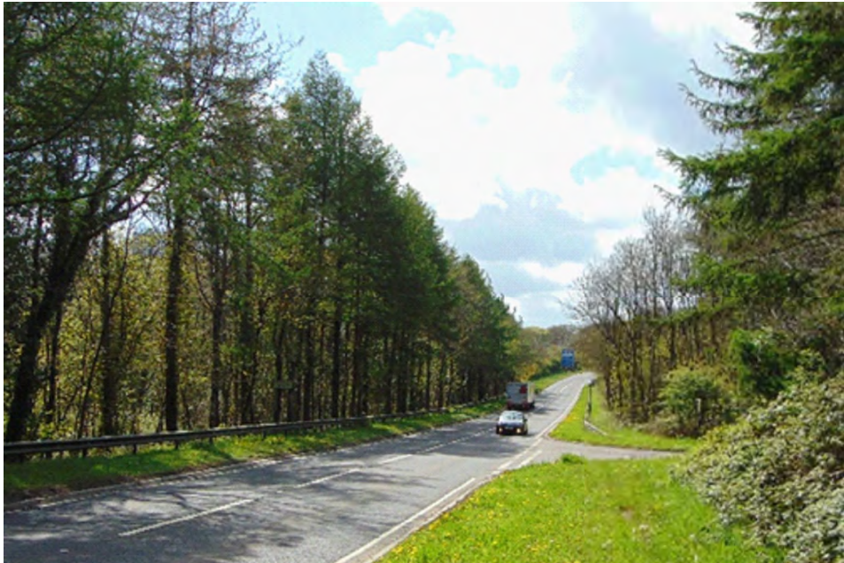
View of the A40 on embankment west through Ffynnon Wood
