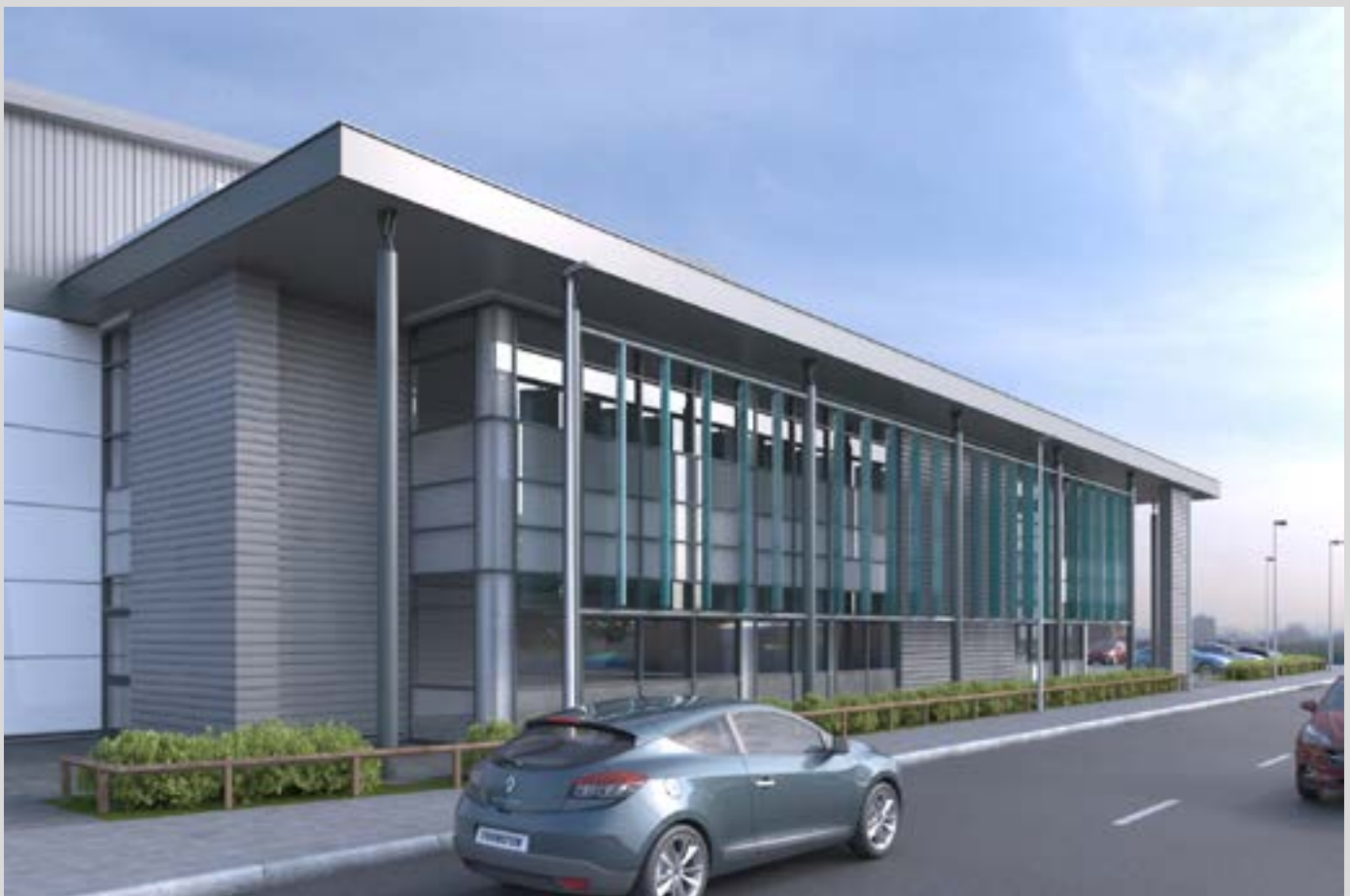
Rhondda Cynon Taf County Borough Council is developing new business premises on the former Coed Ely colliery and coking site
