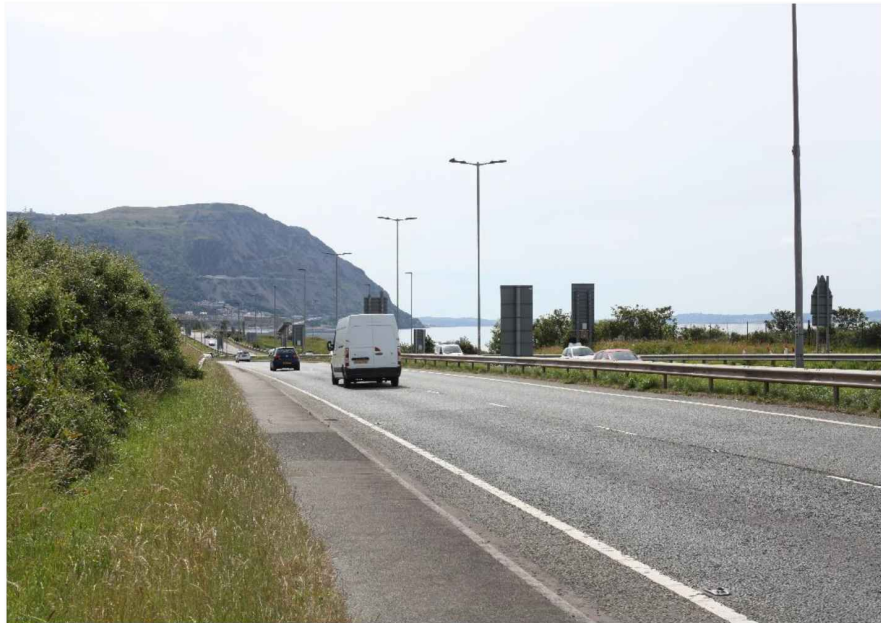
E. A55 westbound carriageway west of Junction 16A.
