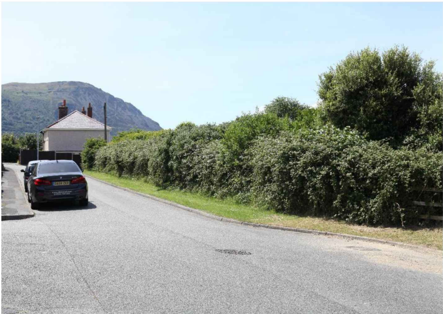
F. Maes-y-Llan residential area to the south of the A55 road corridor.
