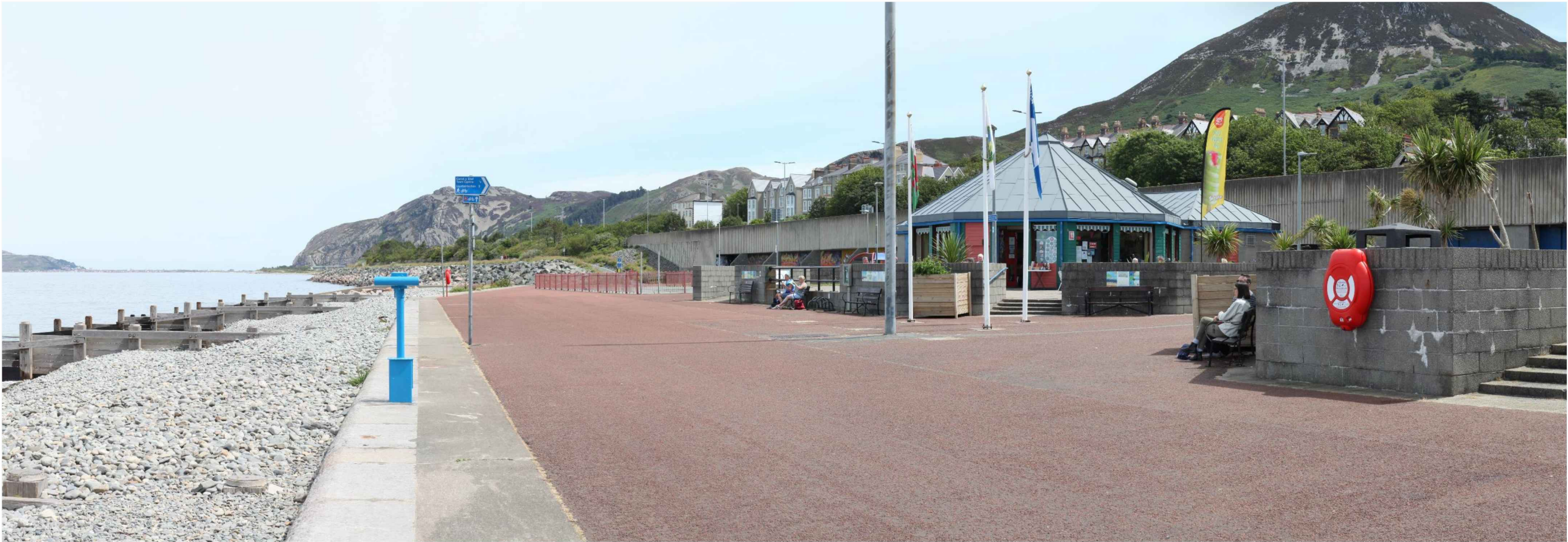
A. View east along Penmaenmawr Promenade with existing A55 road corridor above cafe and play area.
