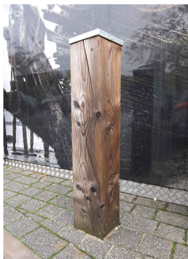
Typical view of timber bollards
