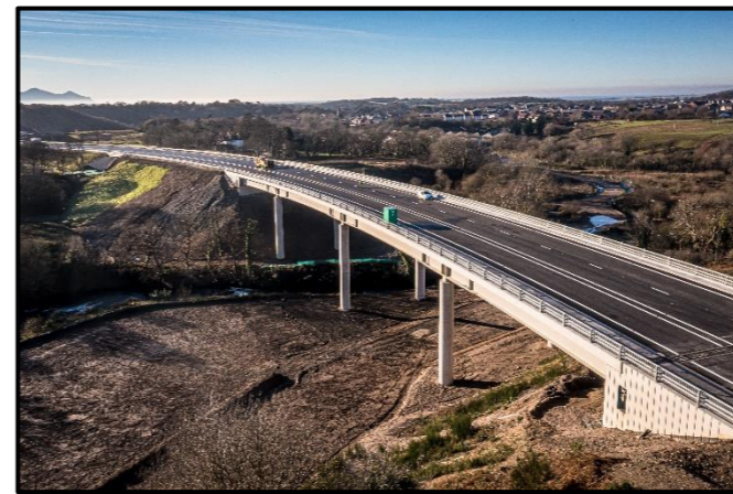
Viaduct over River Seiont
