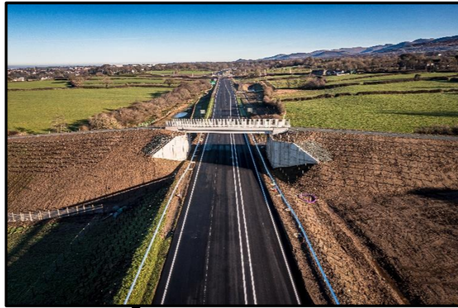
Ceriw Pedestrian/Cycle Bridge
