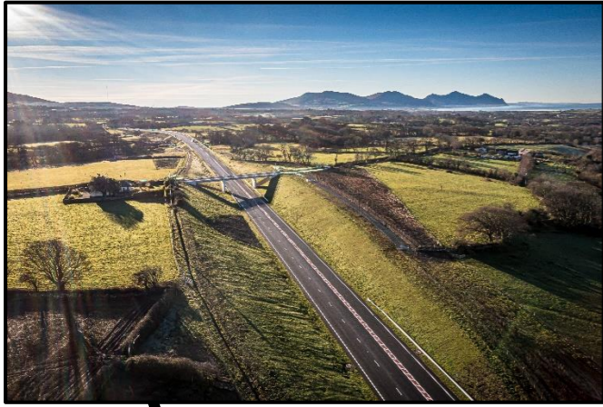
Bridge at Ty'n Llan Road
