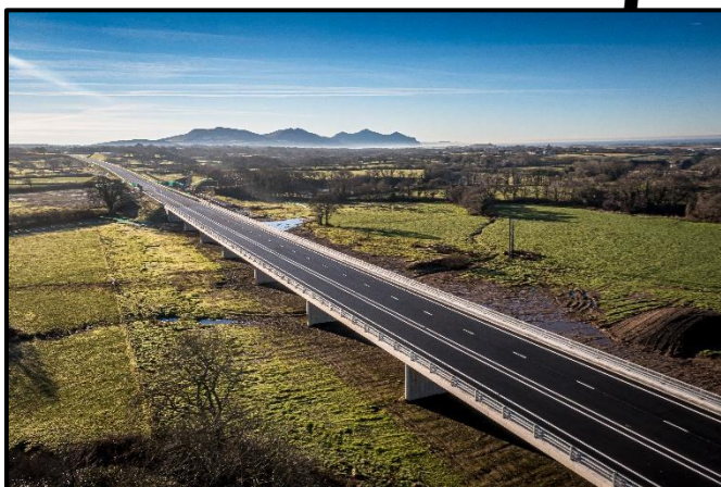
Viaduct over River Gwyrfaï
