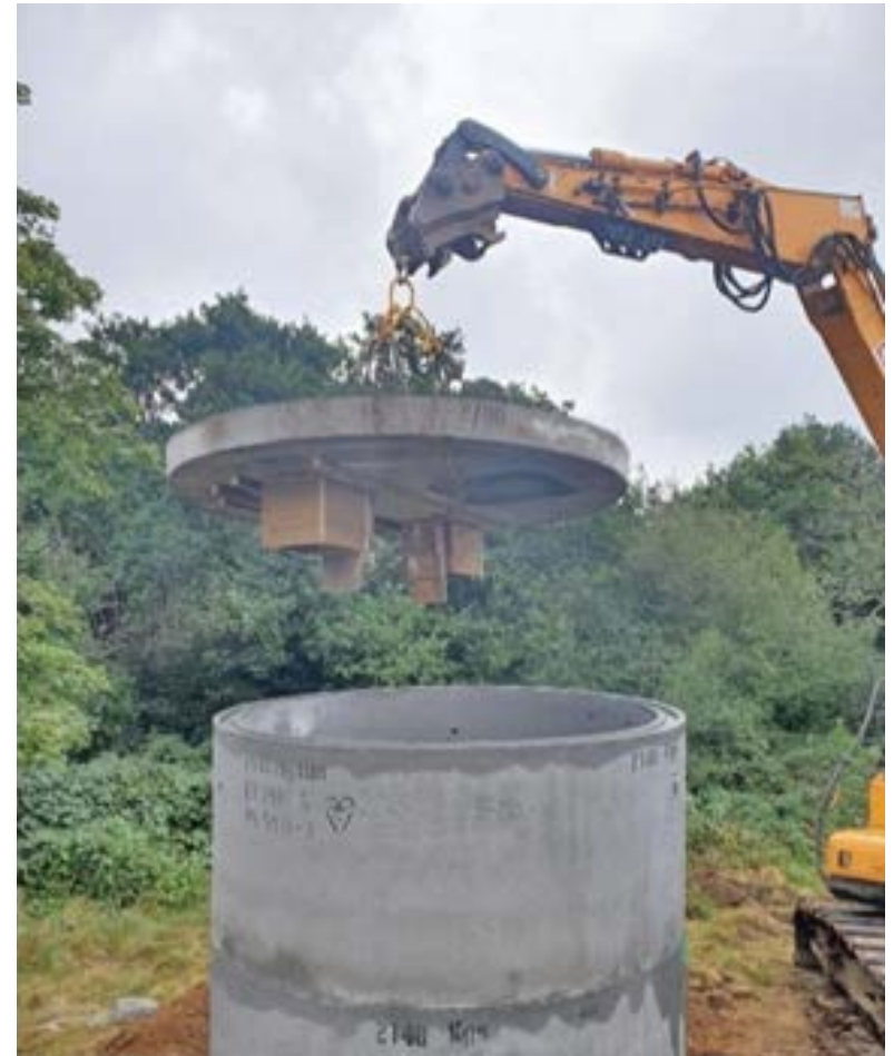
Construction of a replacement bat roost.
