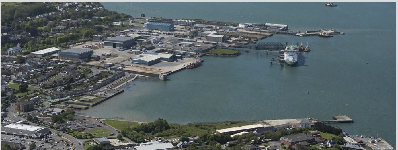
Pembroke Dock Marine project
