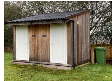
Example of showers / WC's
