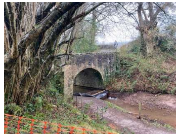
Canal bridge (right of way over)
