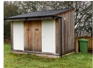
Example of showers / WC's
