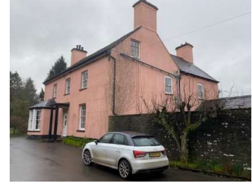
South east and northeast
