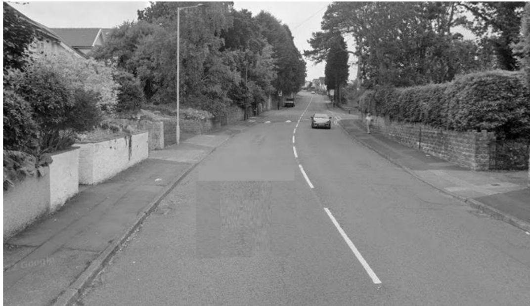
Footway widening to support SUP
