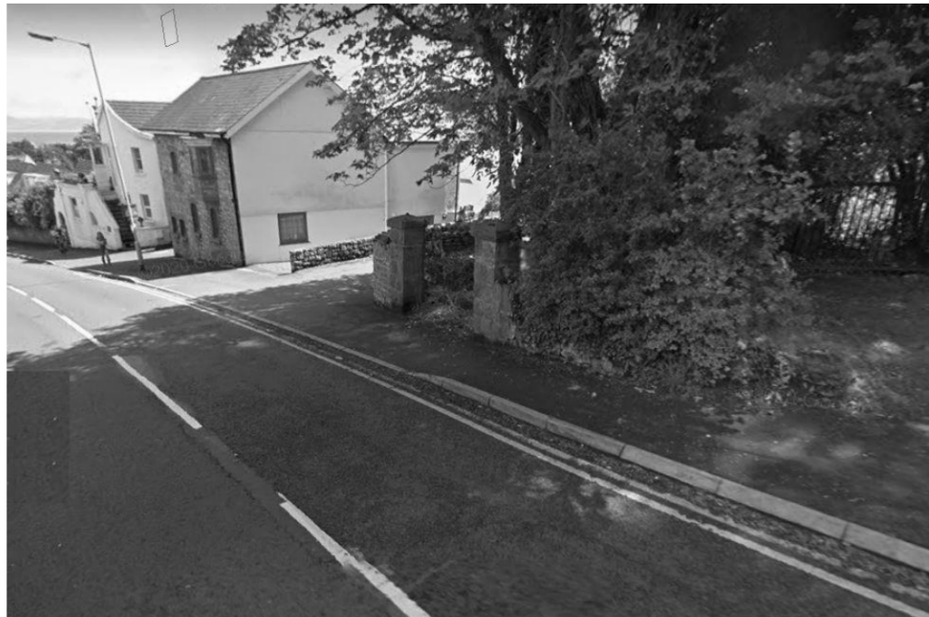
Setting back Wall, Pillars and Railings to support SUP
