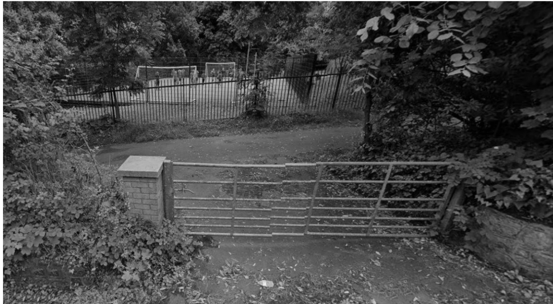
Up grading Existing footway to support SUP
