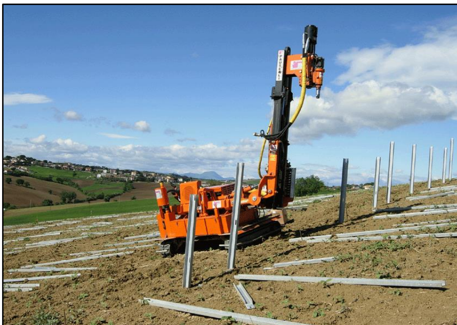
Ffigur 3.7c: Rig gosod pyst sylfaen (o Solar Park Developments)
