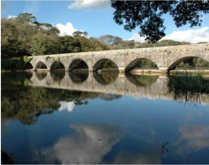
Stackpole bridge credit: Mike May
