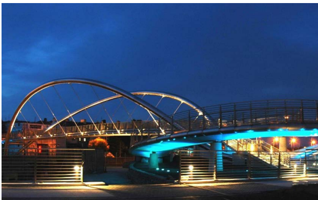
Celtic Gateway Bridge
