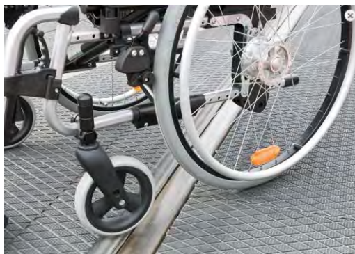
Figure 5-1 – Example of gap filler for street running section 15
