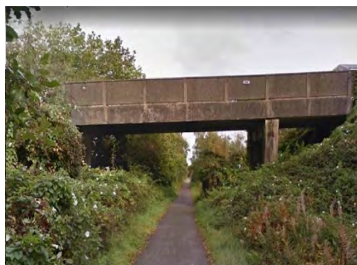
Figure 7-44 – Overbridge crosses alignment Obstruction BC-09-02
