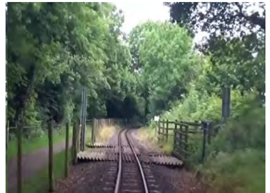
Figure 8-29 – Access track across alignment Obstruction - CD-04-01
