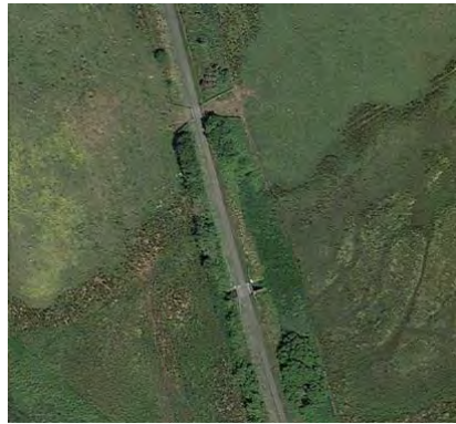
Figure 10-15 – Access Track and Underbridge Obstruction Number – PB-05-03
