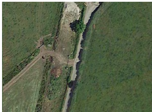
Figure 11-11 – Access track crosses alignment Obstruction - BA-02-06
