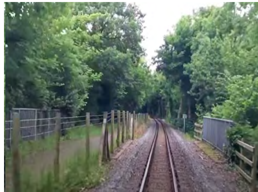
Figure 8-28 – Underbridge over access track Obstruction - CD-03-05
