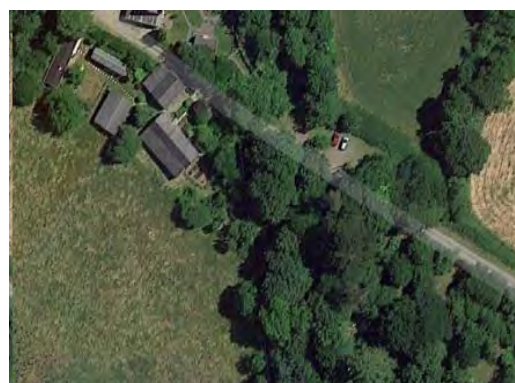
Figure 11-14 – Access track crosses alignment Obstruction – BA-03-03
