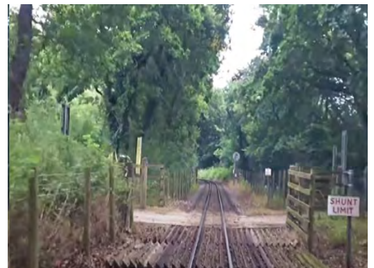
Figure 8-31 – Access track crosses alignment Obstruction - CD-04-03
