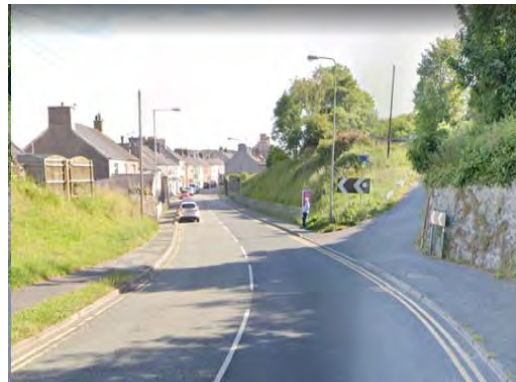
Figure 7-28 – Caernarfon Road crosses alignment Obstruction BC-06-05
