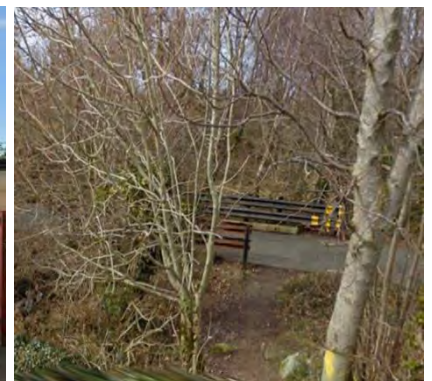
Figure 9-16 – Culvert under alignment Obstruction Number – DP-03-04
