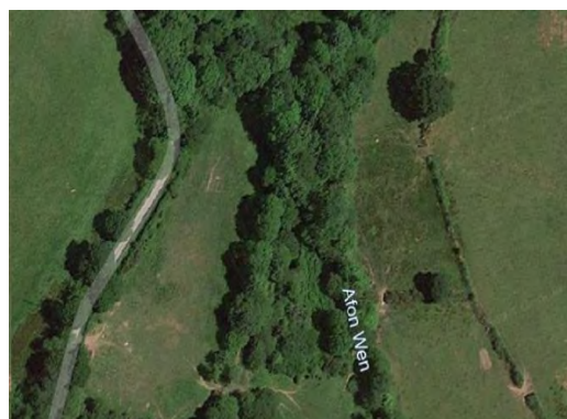
Figure 11-30 – Possible Underbridge Obstruction - BA-06-04
