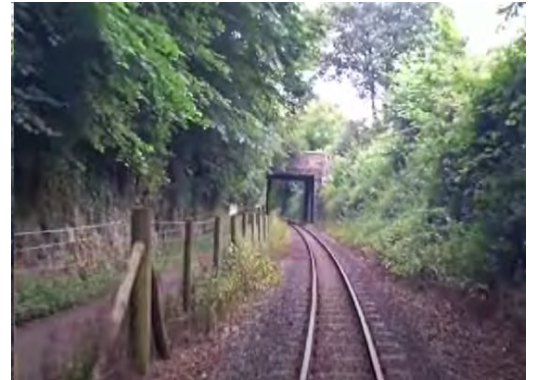
Figure 8-17 – Retaining walls along alignment Obstruction - CD-02-01
