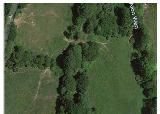
Figure 11-31 – Access track crosses alignment Obstruction – BA-06-05
