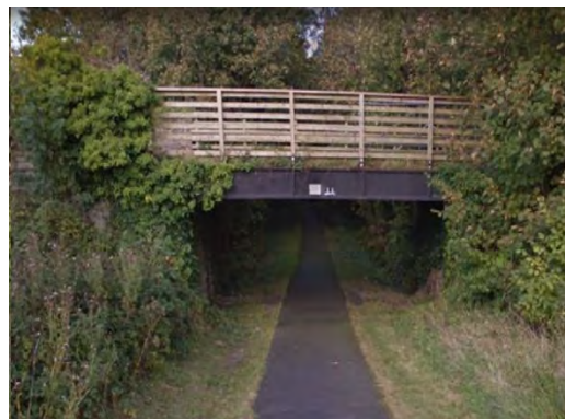
Figure 7-36 – Overbridge crosses alignment Obstruction BC-07-04
