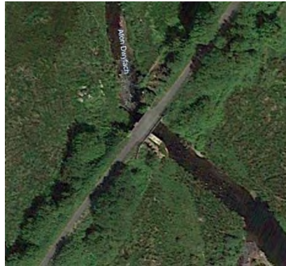
Figure 10-26 – Underbridge over Afon Dwyfach Obstruction Number – PB-07-04
