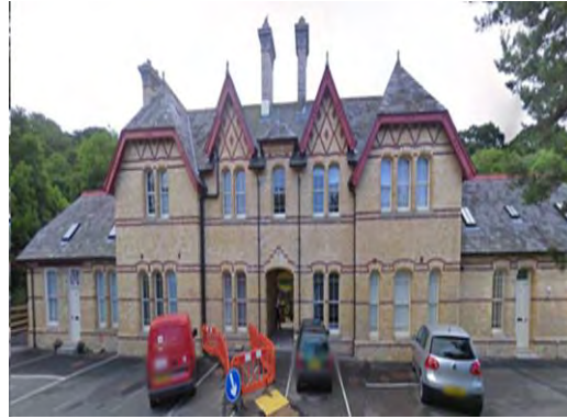
Figure 7-26 – Port Dinorwic Station Obstruction BC-06-04
