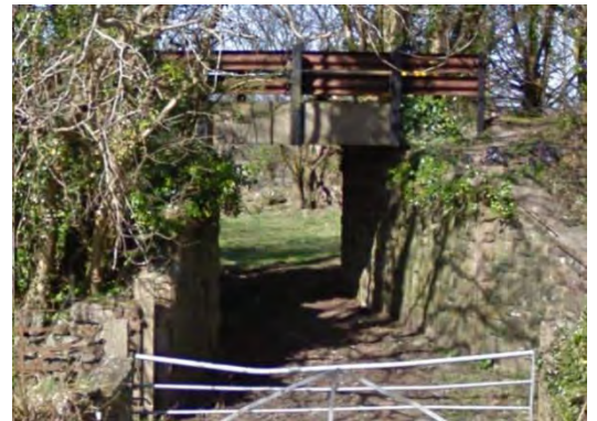
Figure 9-14 – Underbridge over access road Obstruction Number – DP-03-02
