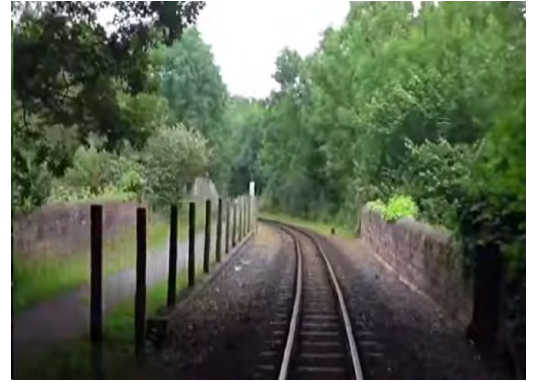
Figure 8-15 – River Seiont Underbridge Obstruction - CD-01-07
