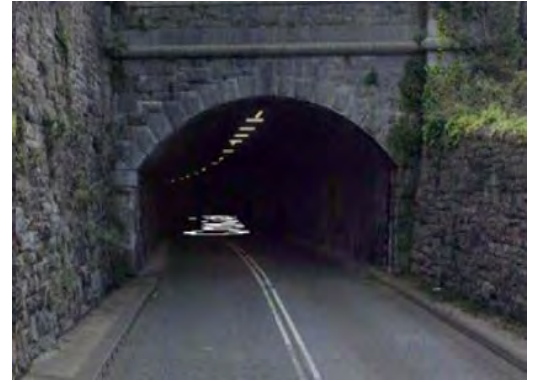
Figure 7-57 – Tunnel along alignment Obstruction BC-11-08
