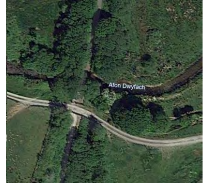
Figure 10-27 – Underbridge over Afon Dwyfach Obstruction Number – PB-08-01
