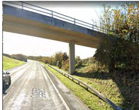
Figure 10-9 – Overbridge crosses alignment Obstruction Number – PB-02-04
