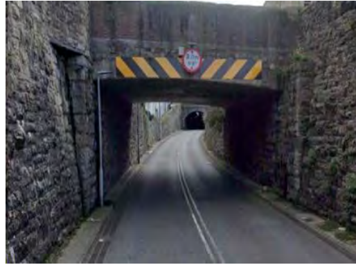
Figure 7-56 – Overbridge crosses alignment Obstruction BC-11-07
