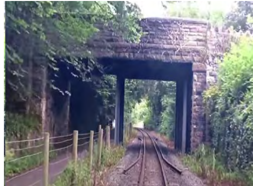
Figure 8-16 – Overbridge carrying Coed Helen Lane Obstruction - CD-01-08
