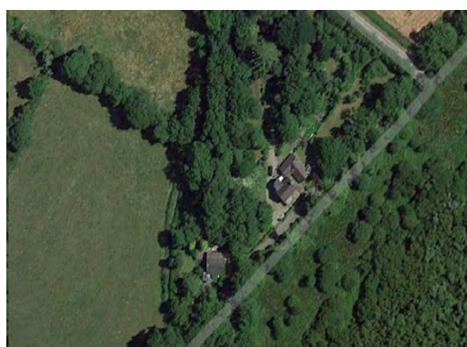
Figure 11-15 – Road crosses alignment Obstruction - BA-03-04
