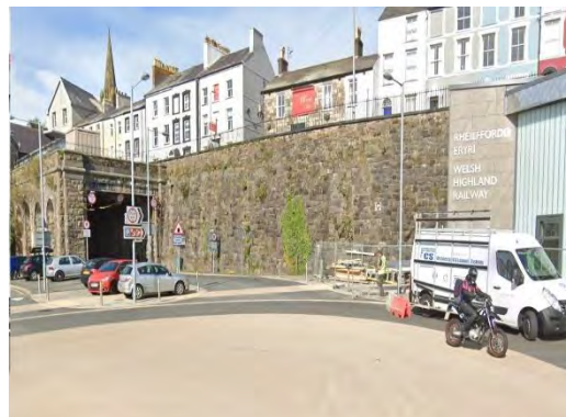
Figure 8-2 – South Portal of Caernarfon Tunnel
