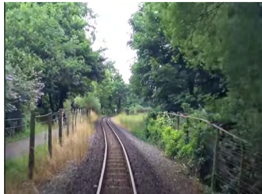
Figure 8-10 – Potential underbridge Obstruction - CD-01-04
