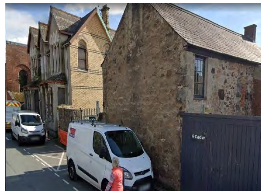
Figure 8-5 – Two listed building on St Helens Road
