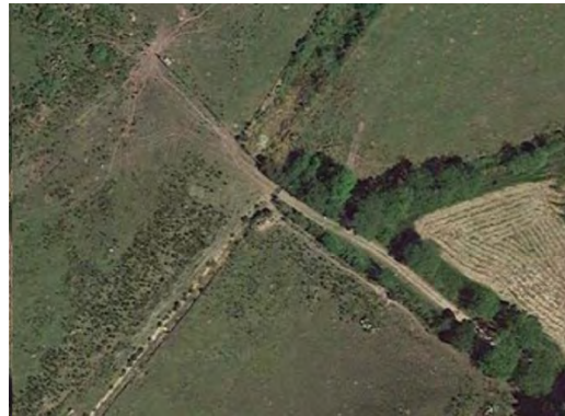
Figure 11-28 – Access track crosses alignment Obstruction - BA-06-02
