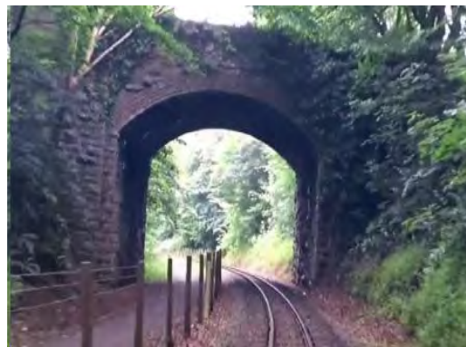
Figure 8-30 – Overbridge crosses alignment Obstruction - CD-04-02
