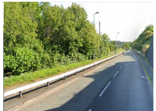
Figure 7-31 – Alignment taken by road Obstruction BC-06-07
