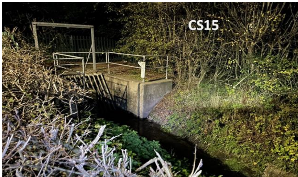
Figure D.3: Chester Road East - Trash Screen
