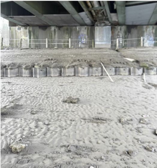
Figure 4.6: Mid and upper littoral underneath the existing bridge (south side)
