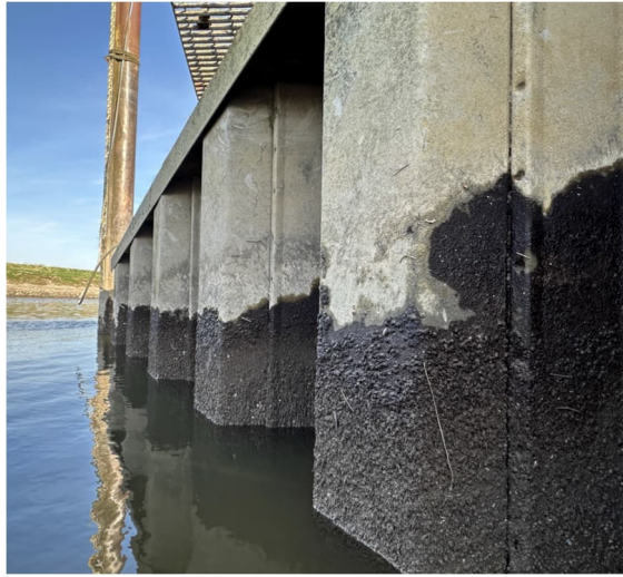
Figure 4.19: Sheet piles encompassing the ALOF
