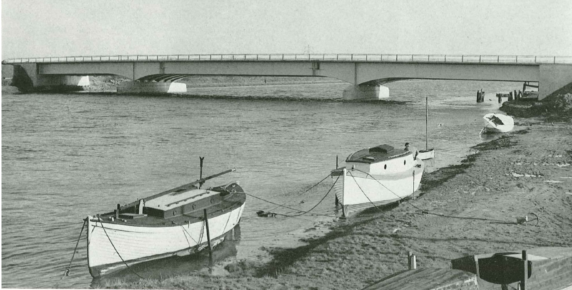
Figure 17 The new River Bridge (Mott Hay and Anderson, 1962). Note extensive evidence of landing stages site 51, east of the arch. View to east.
