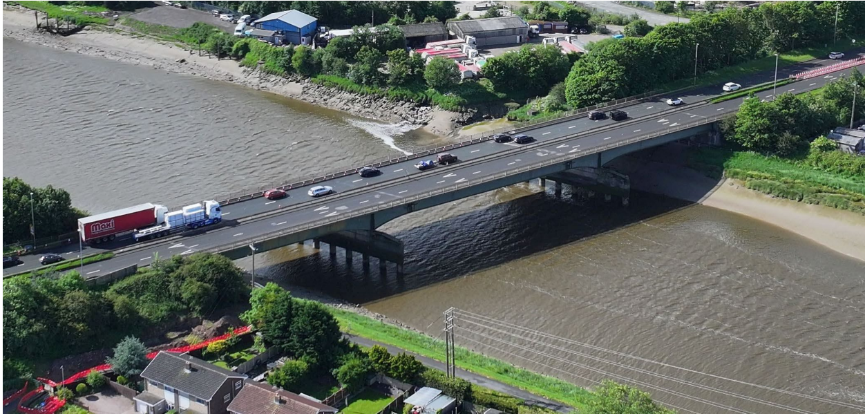
Figure 19. Drone image of the A494 Queensferry bridge, June 2024, from a similar viewpoint to the 1962 Figure 18. View to southeast.
