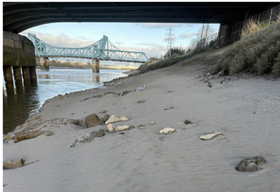
Figure 4.12: Intertidal area below the existing bridge structure
