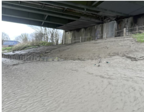
Figure 4.7: Upper littoral showing mud between saltmarsh under existing bridge
