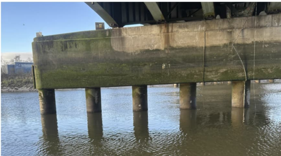
Figure 4.13: Tubular green and filamentous brown algae on north side of existing bridge structure
