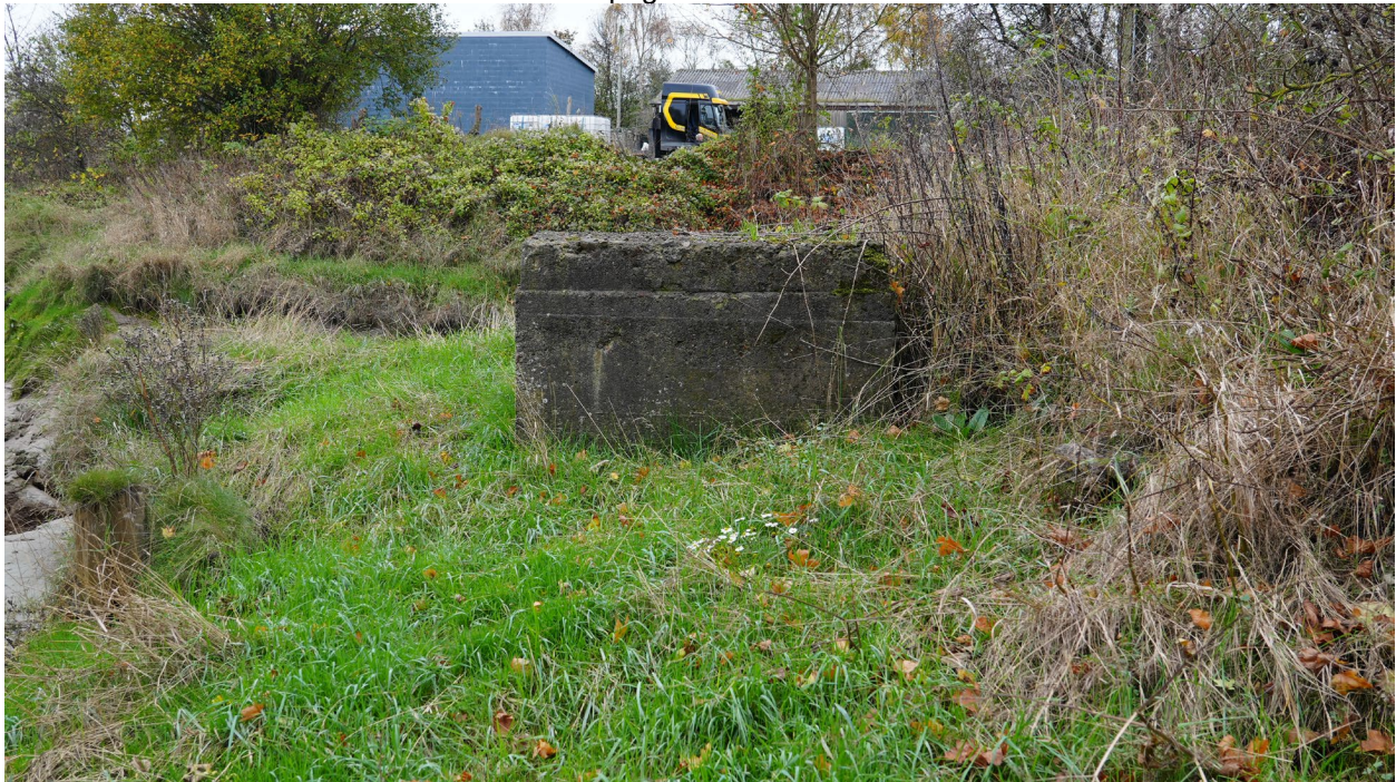
Figure 24 Site 51 concrete block and timber upright to the left. View to the east.
