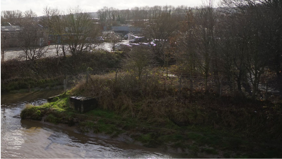
Figure 21 Detail of landing stage (51). Timbers can be seen at the water's edge with two concrete blocks above. A further concrete block is visible in the undergrowth beyond the fence. The fourth block visible in 1962 cannot be seen. View to south.
