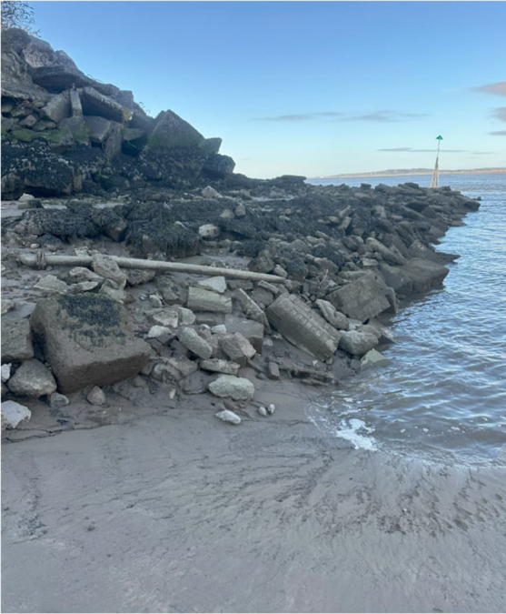
Figure 4.35: Groyne in west end
