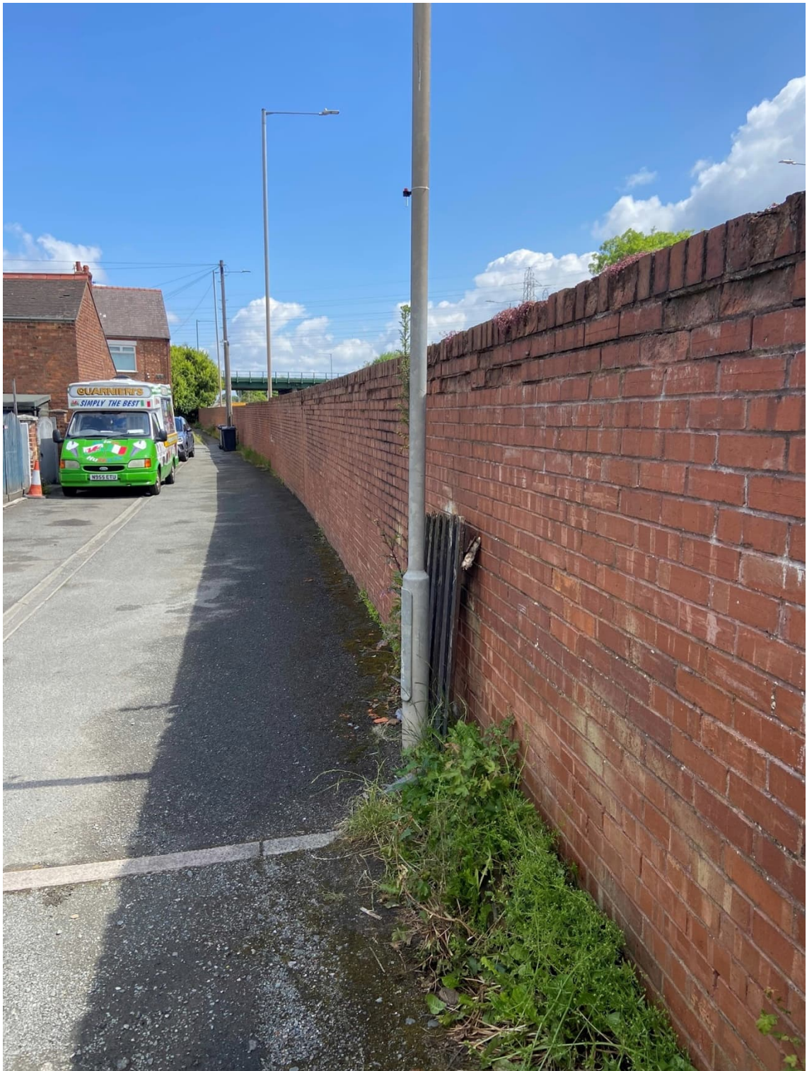
Figure C-2 Photo of diffusion tubes installed at Site D2
