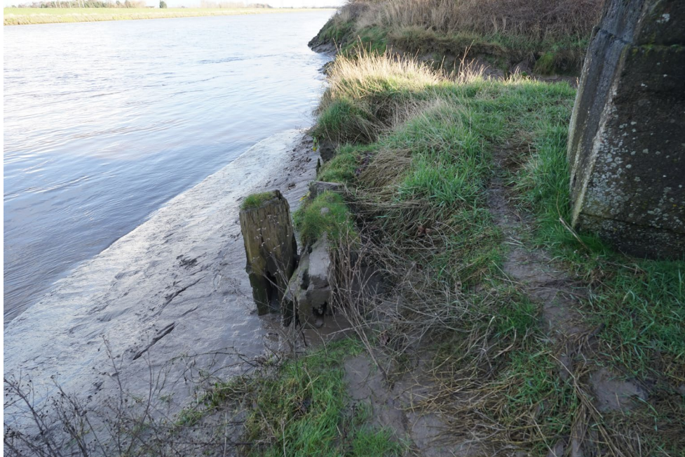
Figure 26 Site 51. Detail of timbers and concrete block. View to east.
