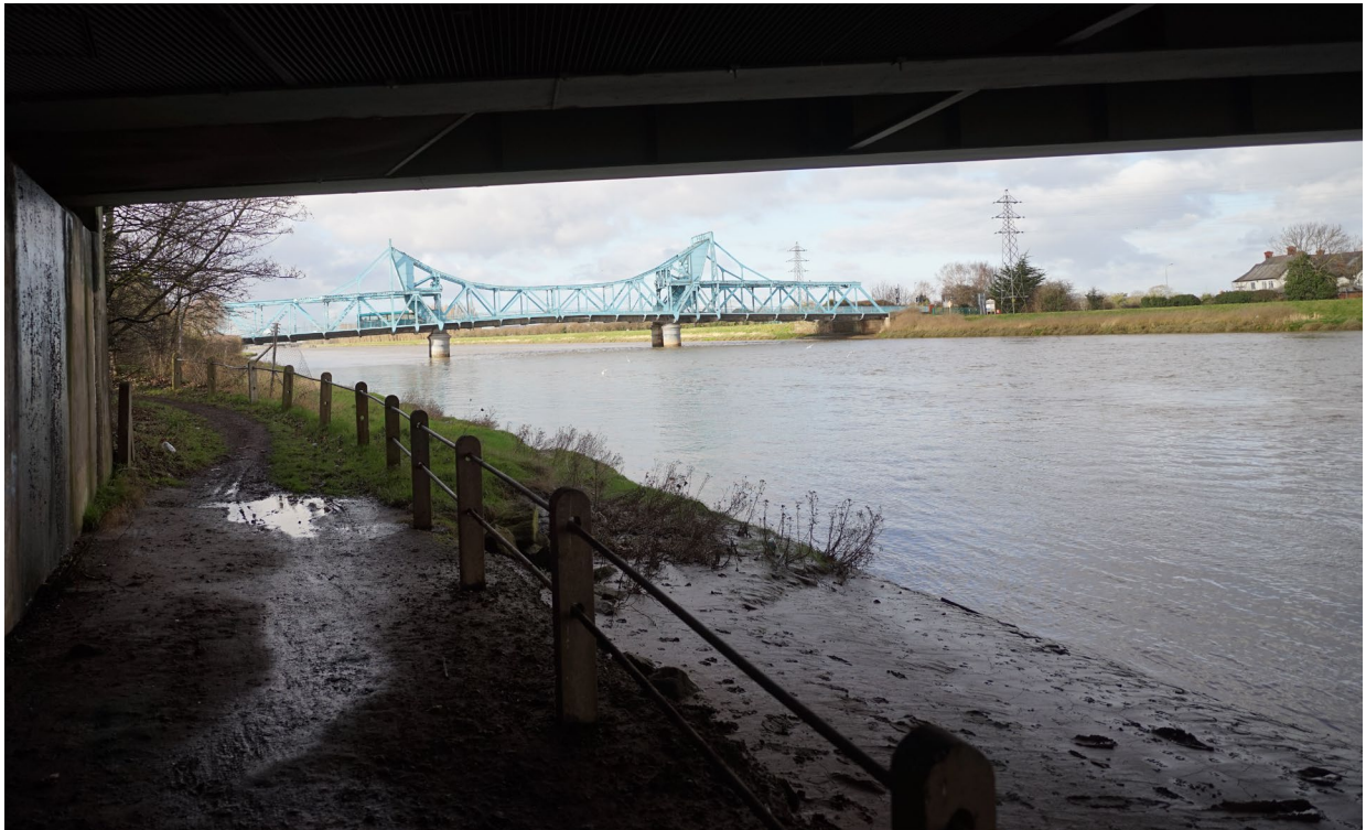
Figure 16 Site 31. Bascule Bridge viewed from under existing Dee Bridge. View to northwest.
