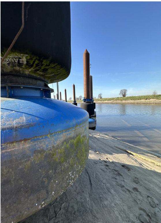
Figure 4.22: Fenders extending to the lower littoral, facing northwest
