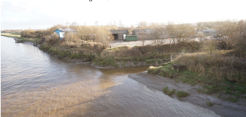
Figure 20 Landing Stage sites 51, 53, 55 and 57. Compare this view with that in 1962 (Figure 18). No evidence for 53 is visible. All have suffered some damage since 1962. View to southeast.
