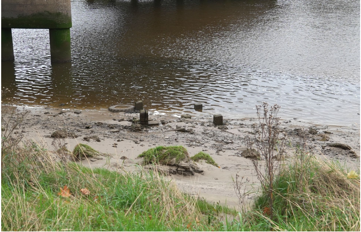
Figure 27 Site 51 concrete post bases. View to the north.
