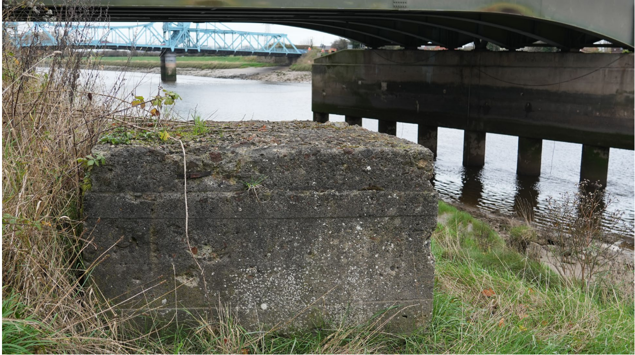
Figure 25 Site 51 concrete block with Site 33 Jubilee Bridge to rear. View to northwest.
