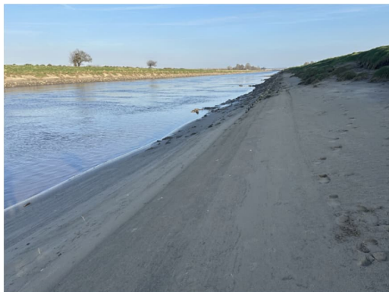
Figure 4.21: Area east of the ALOF site, facing east
