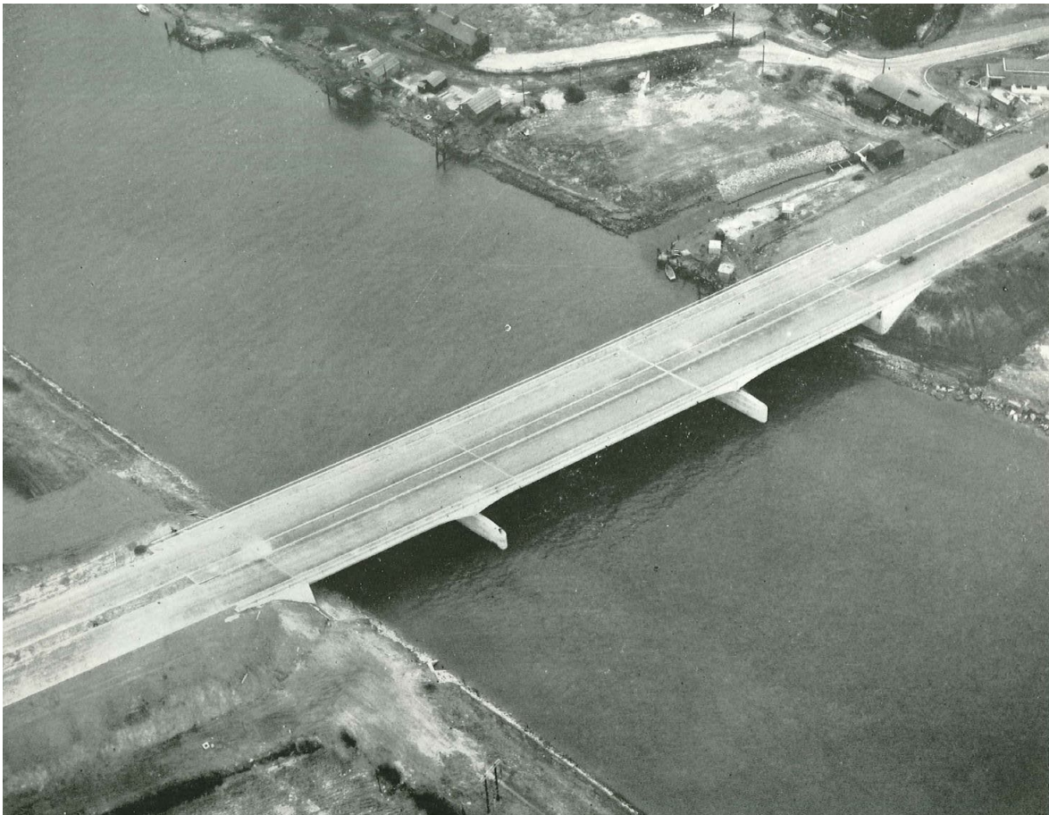
Figure 18 An Aerial Photograph of the New Bridge (Mott Hay and Anderson, 1962). Landing stage sites 51, 53, 55 and 57 are clearly visible. Note the extent of work around the Aston Inlet, Aston Shipyard (48) and Aston Quay building (43).
