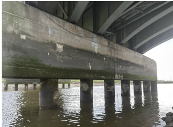
Figure 4.14: South side of existing bridge structure
