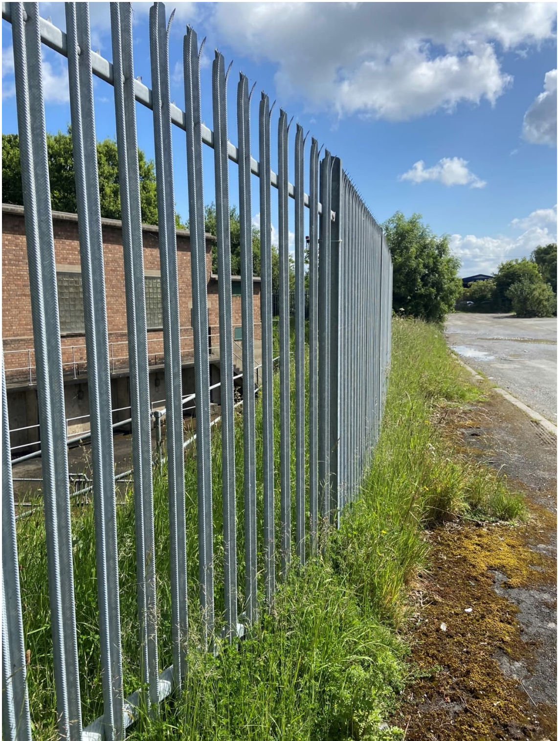
Figure C-6 Photo of diffusion tubes installed at Site D6
