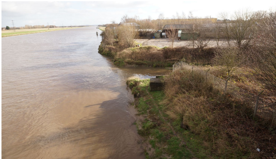
Figure 22 Sites 51, 55 and 57. Surviving structures. View to east.
