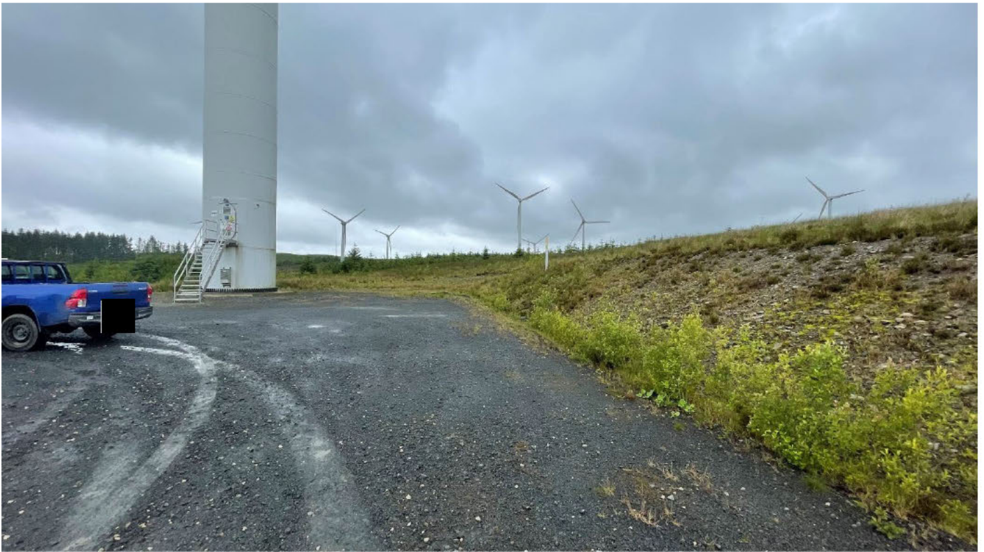
Above (looking north west) and below (looking south east), images of excavated turbine blade laydown pad and crane pad at https://what3words.com/bleaker.should.tributes
