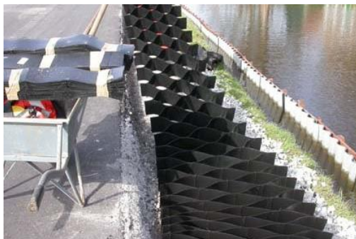
Image 3 – Geocell Containment System
