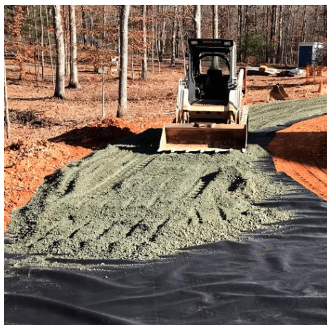
Image 1 - Fabric Separation layer
