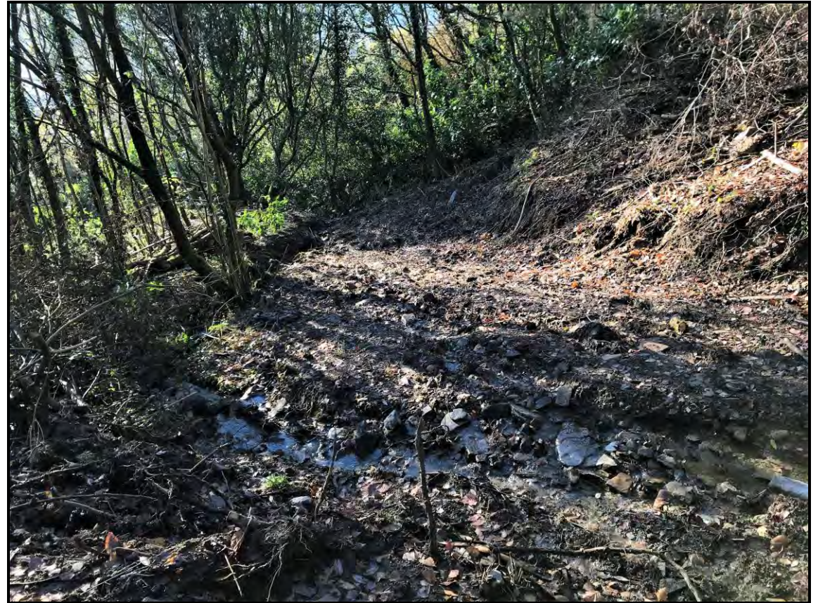
Plate 16: Looking downslope to the west, saturated ground with streams flowing from base of spoil tip.
