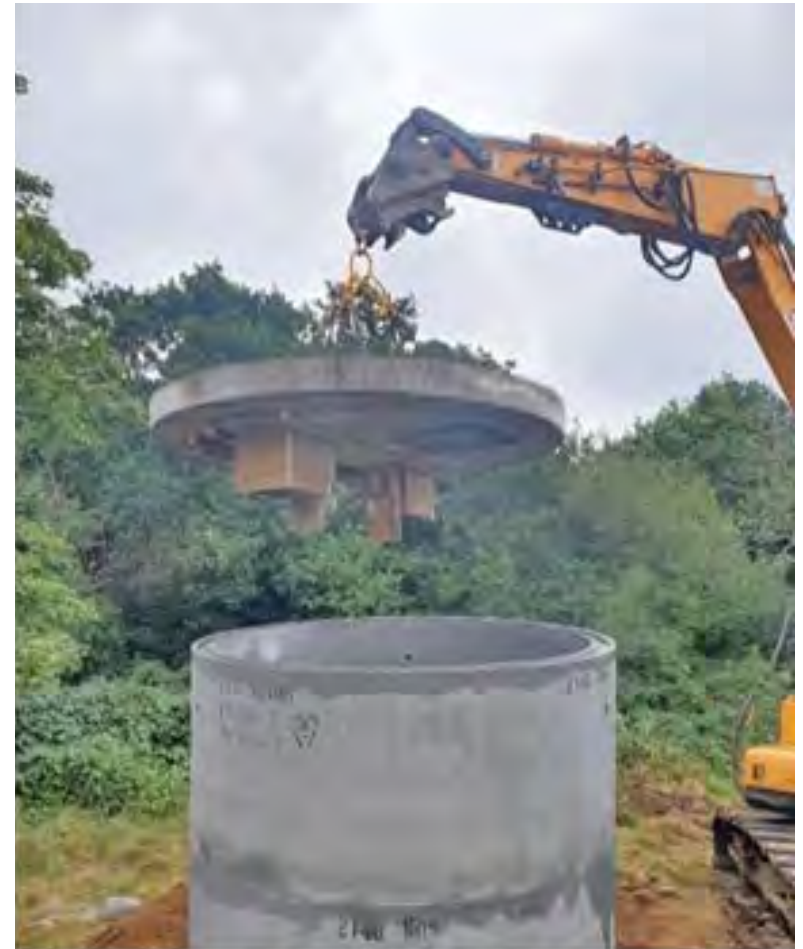
Construction of a replacement bat roost.
