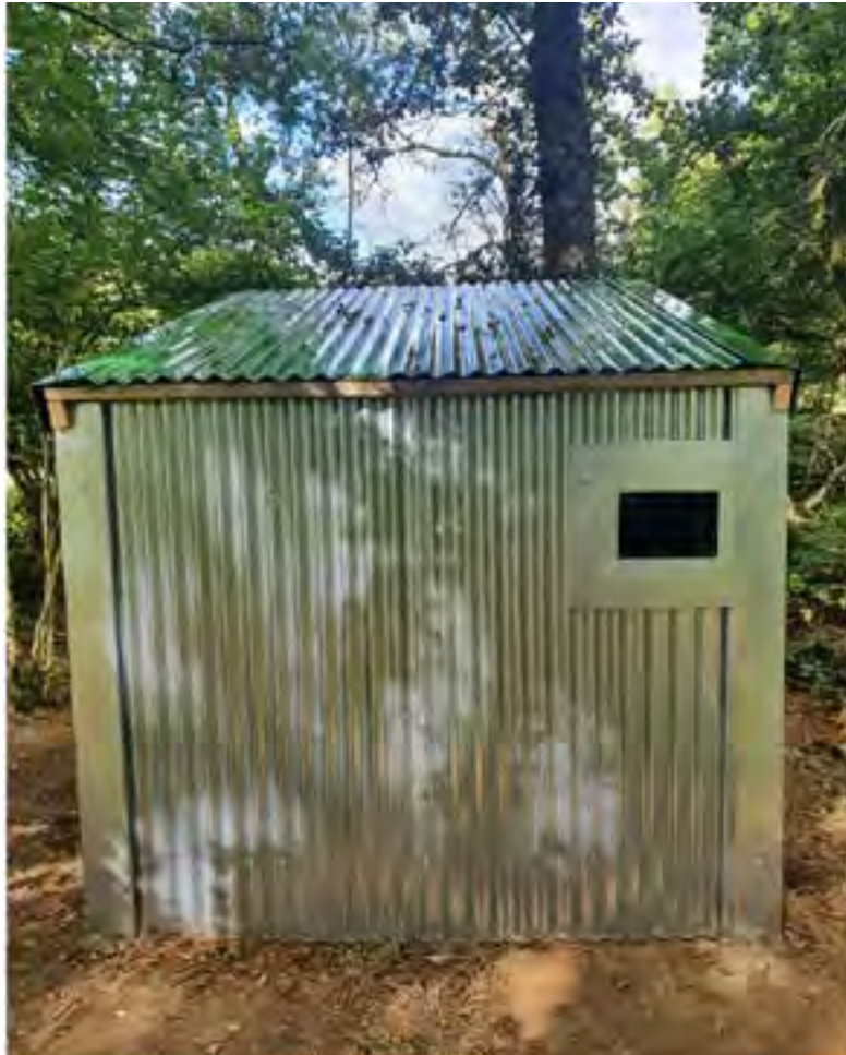
Replacement bat roost.
