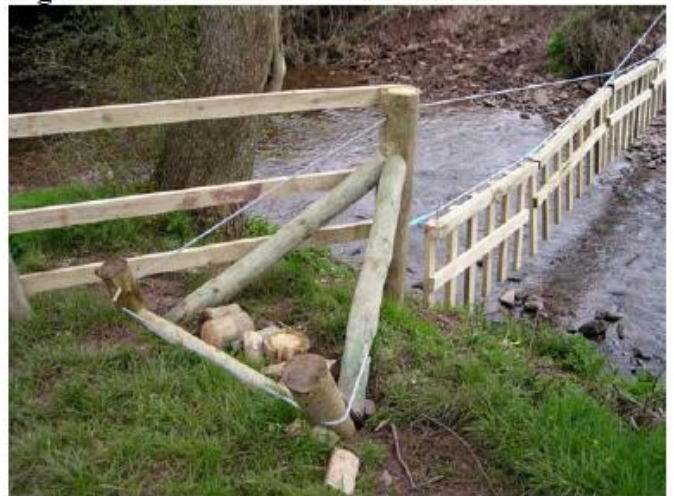
Figure 4: Good anchor & cantilever
