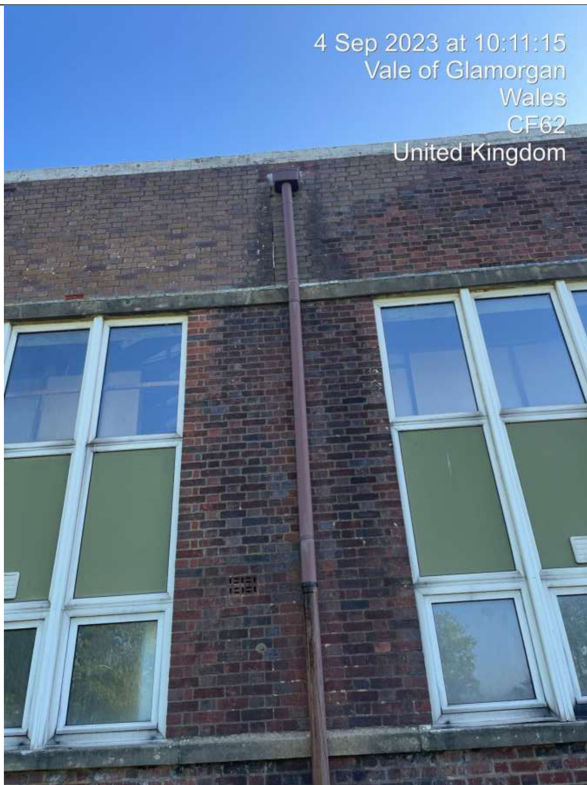
Western Elevation. Downpipe from Hidden Gutter.
