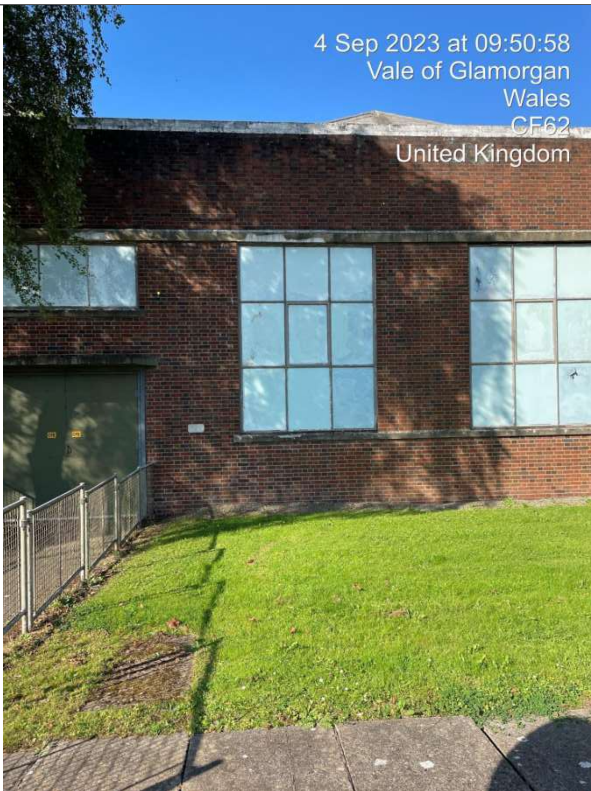
Eastern Elevation. Original Fenestration.
