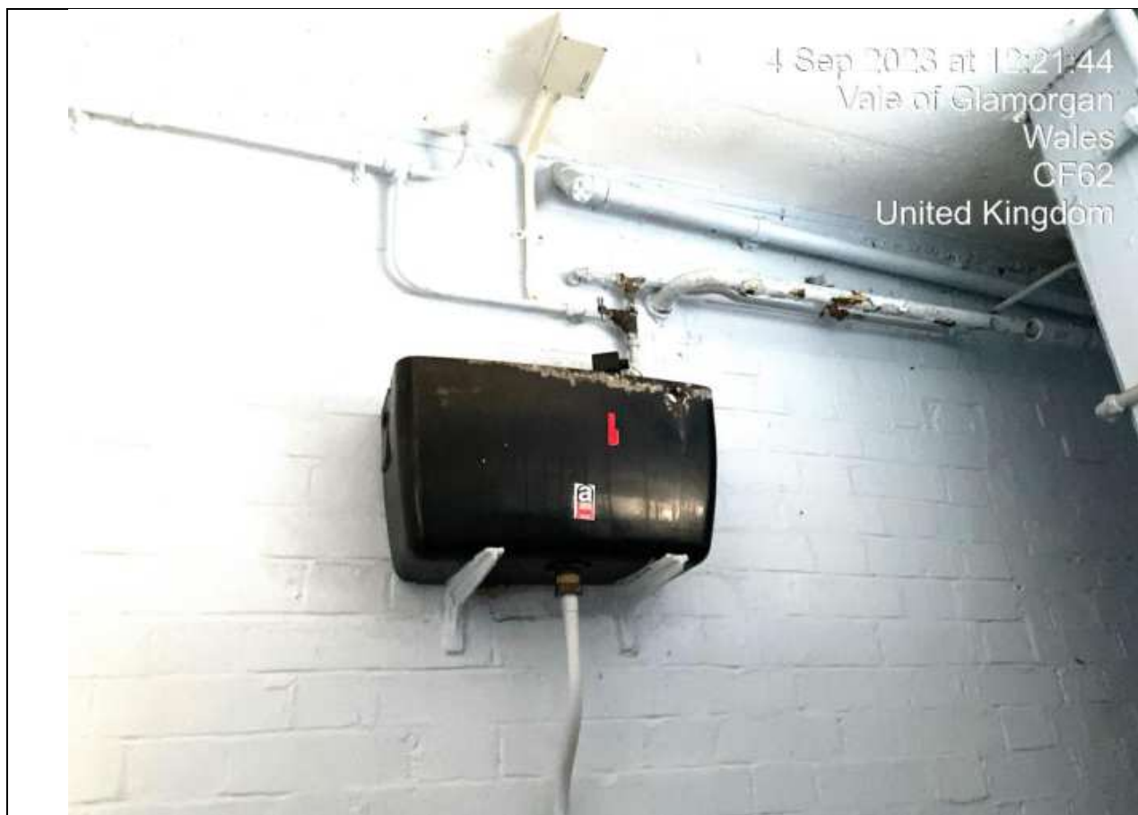
Asbestos Content to High Level Toilet Cistern.
