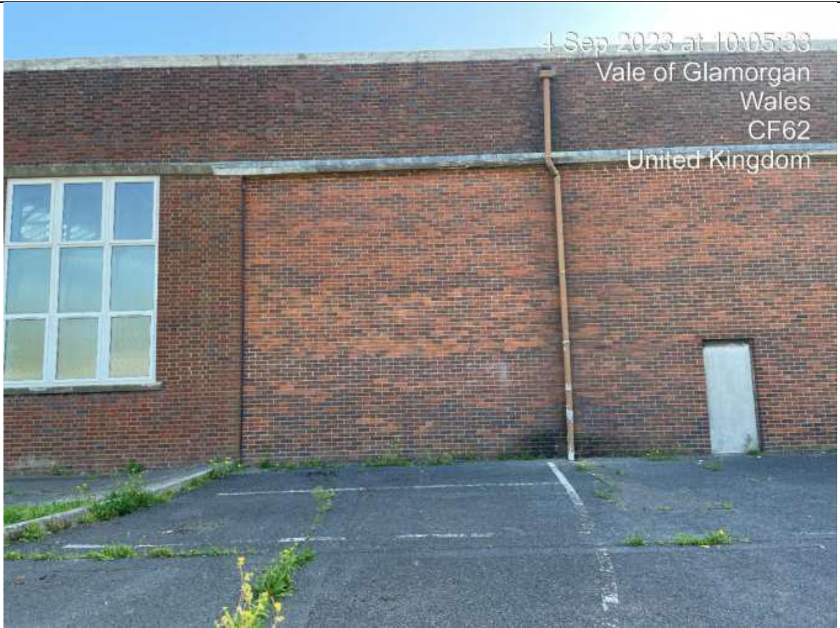
Western Elevation. Bricked-Up Original Entrance Way.
