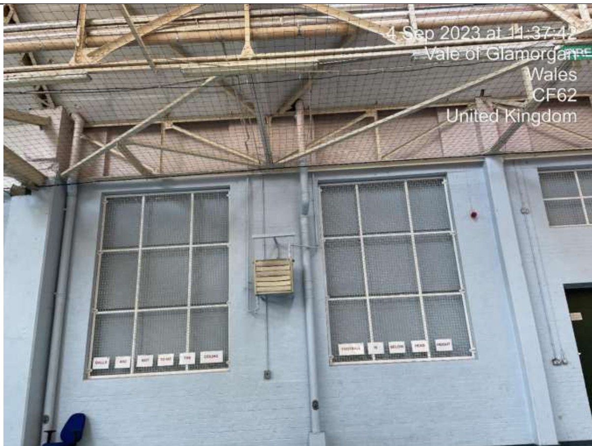
Covered Original Fenestration.
