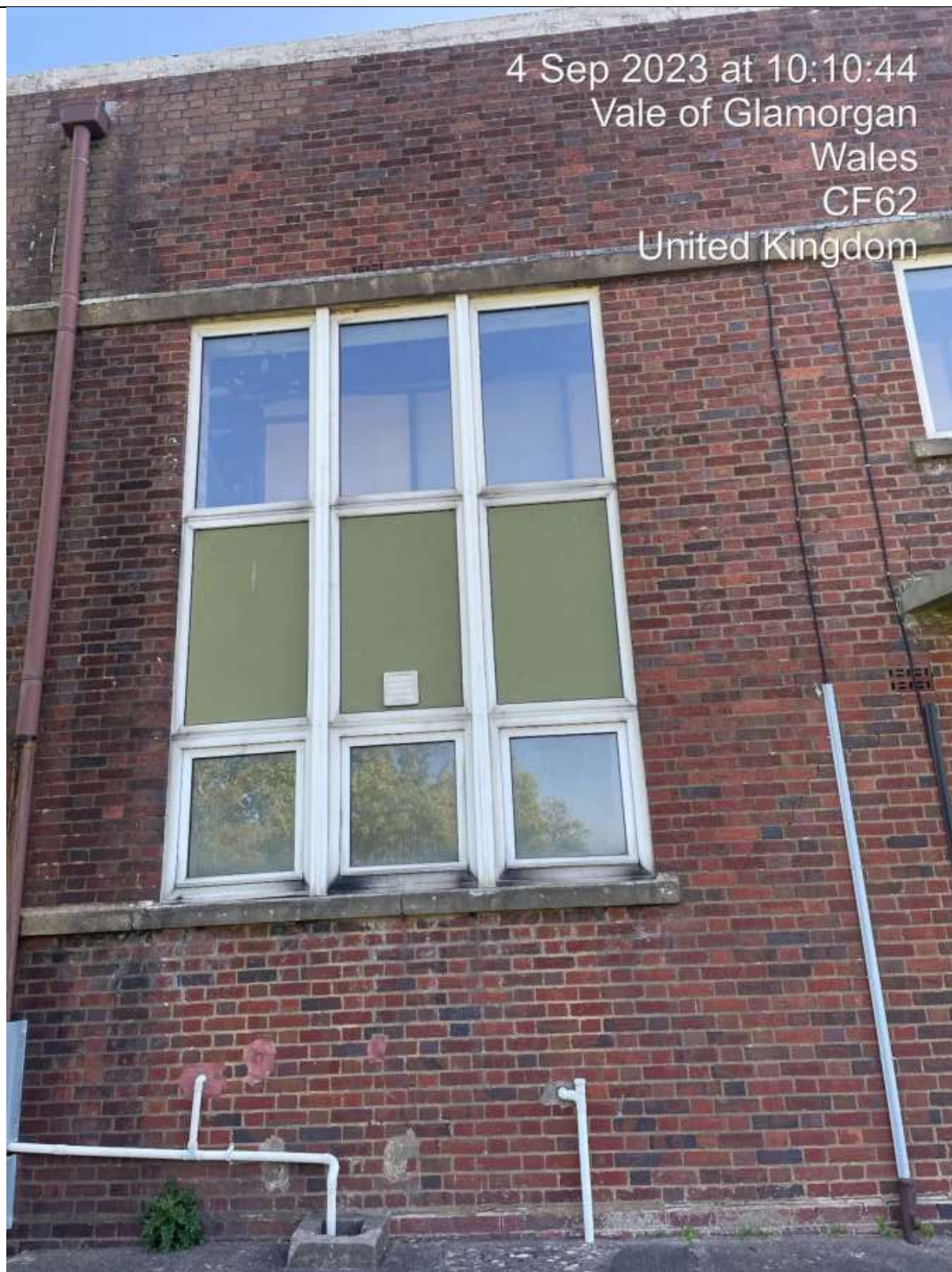
Western Elevation. Replacement Fenestration.
