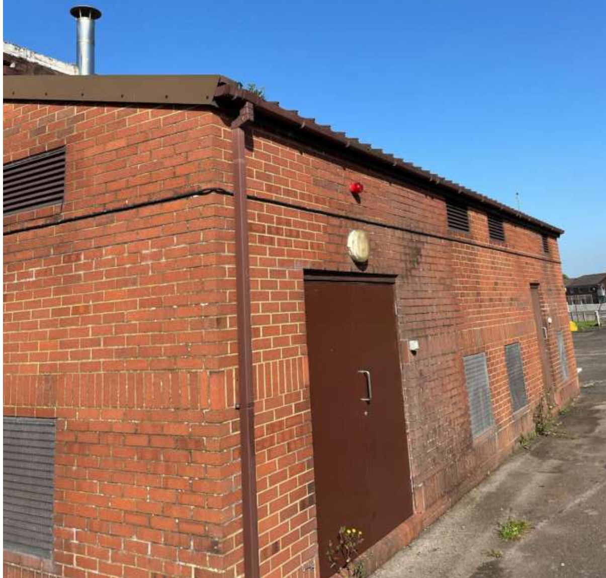
Eastern Elevation. Non-Original Plant Room Addition.
