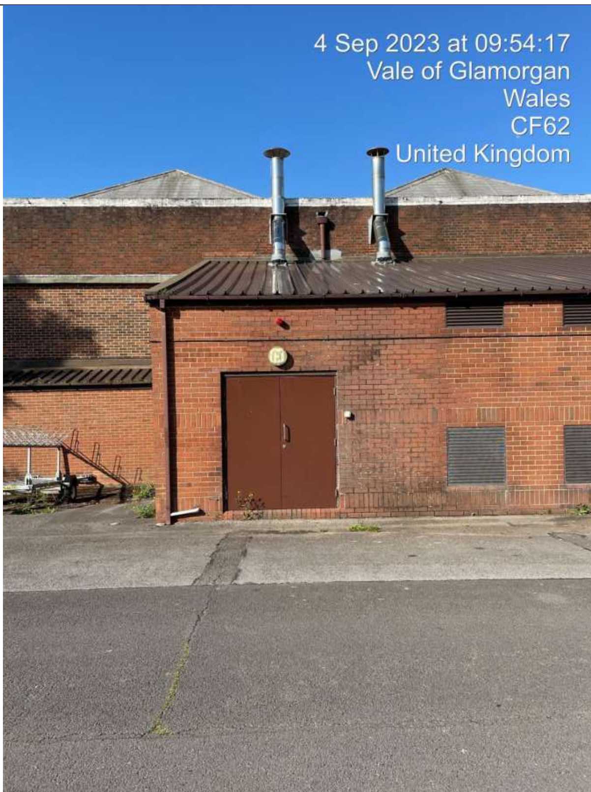
Eastern Elevation. Non-Original Plant Room Addition.
