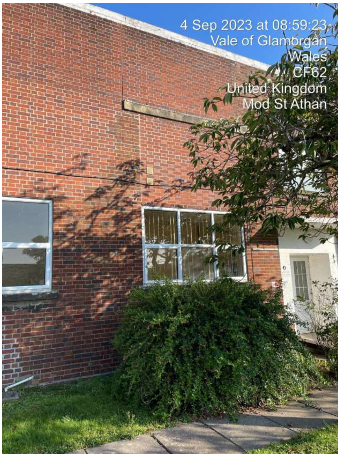
Southern Elevation. Note the Replacement Brickwork & Replacement Fenestration.
