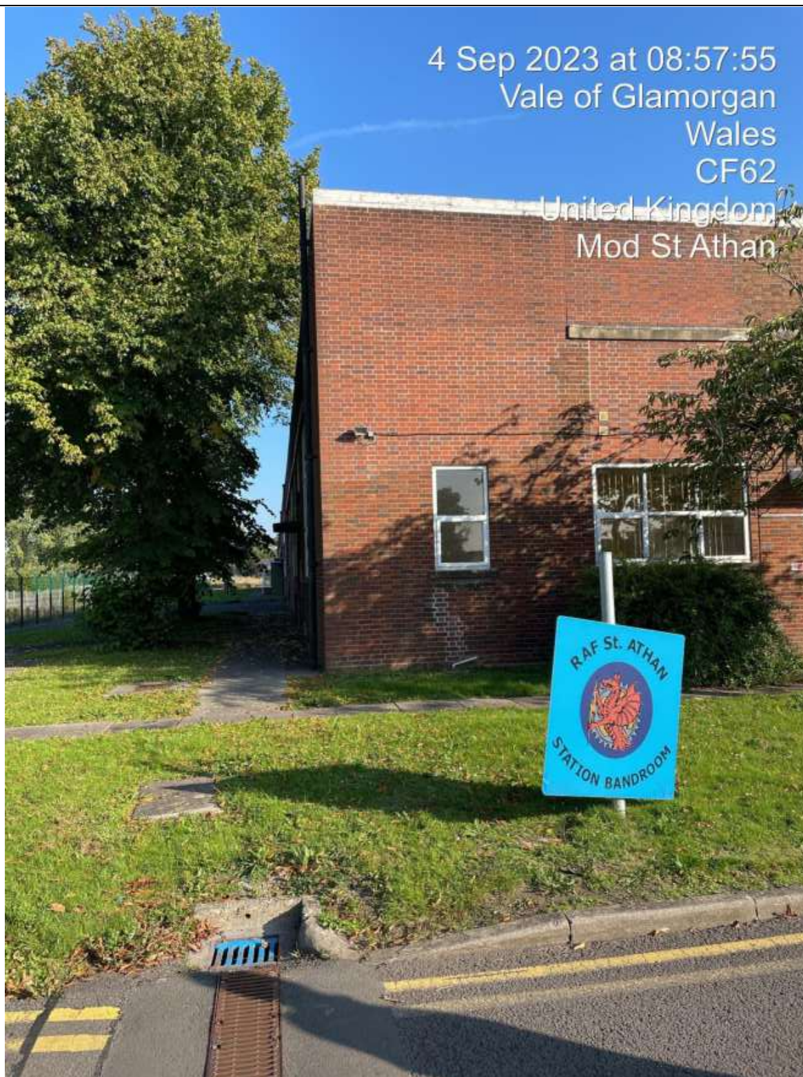
Corner of Southern & Western Elevations. Note the Replacement Brickwork & Replacement Fenestration
