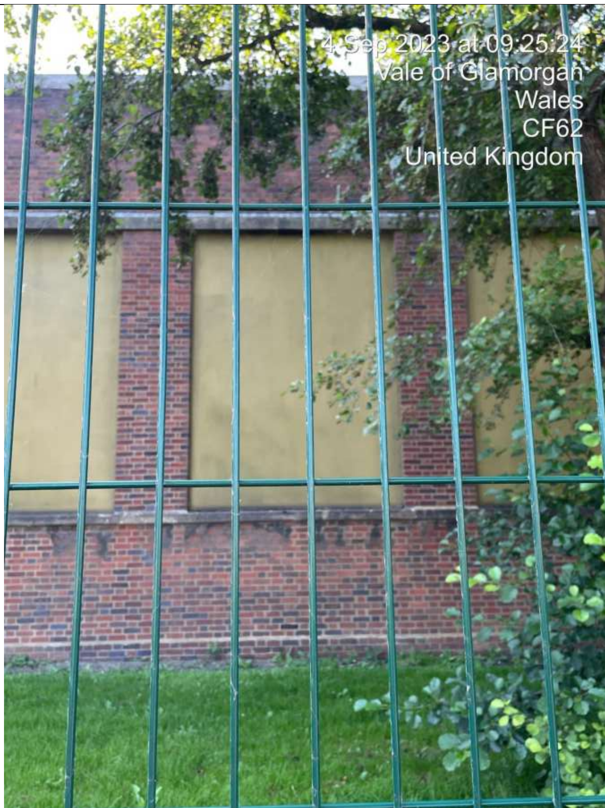
Northern Elevation. Blanked Off Fenestration.
