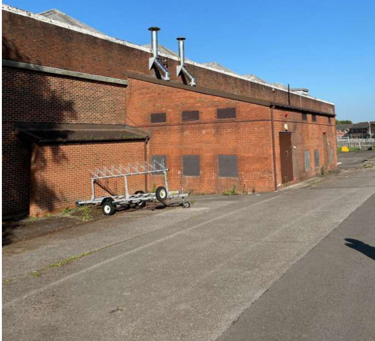
Eastern Elevation. Non-Original Plant Room Addition.
