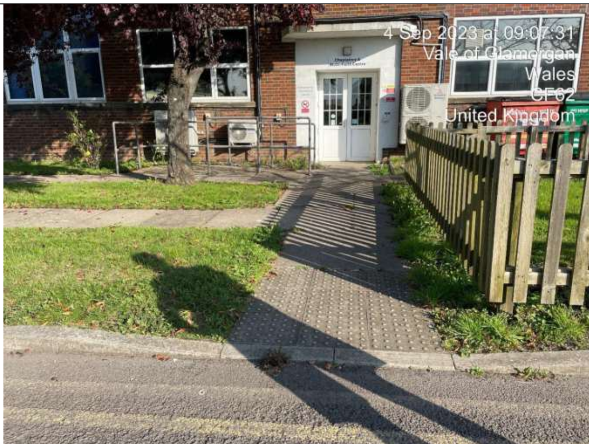
Southern Elevation. Non-Compliant Entrance to Chaplaincy & Multi-Faith Centre.
