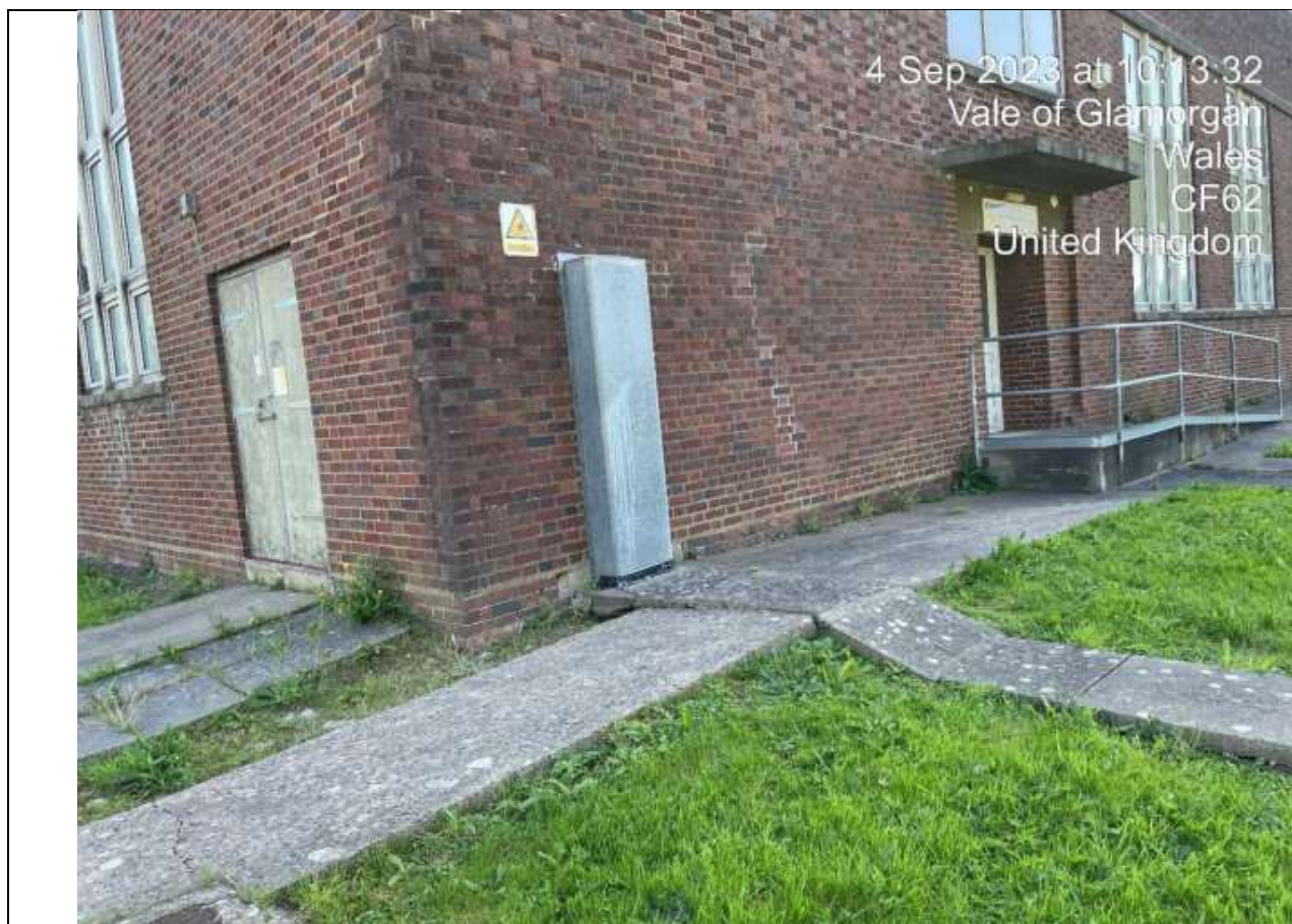
Western Elevation. Significant Electrical Services Point of Penetration.
