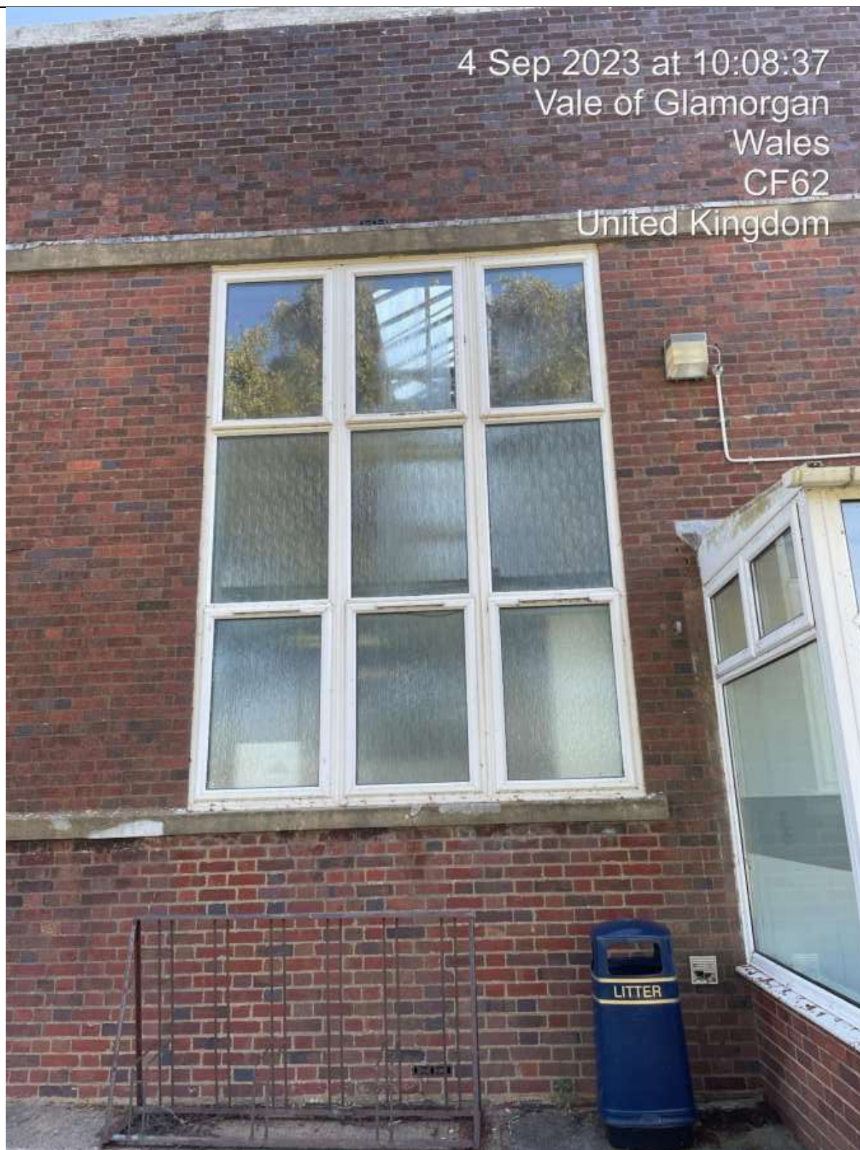
Western Elevation. Replacement Fenestration.
