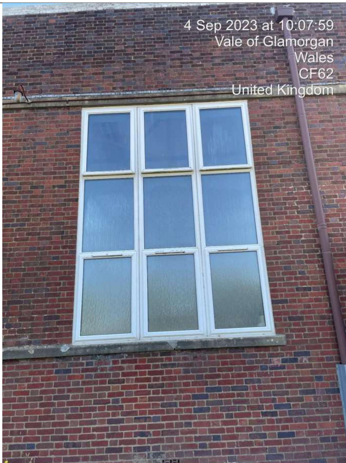
Western Elevation. Replacement Fenestration.
