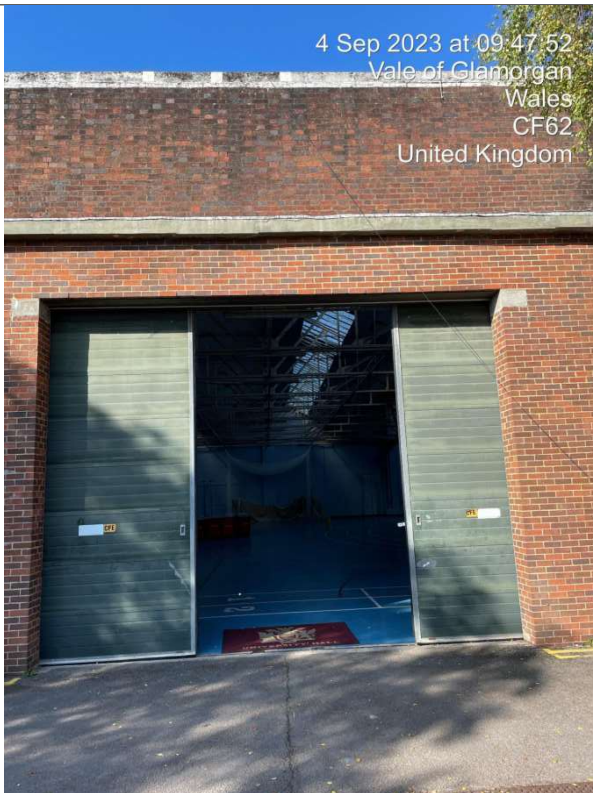
Eastern Elevation. Modified Entrance.
