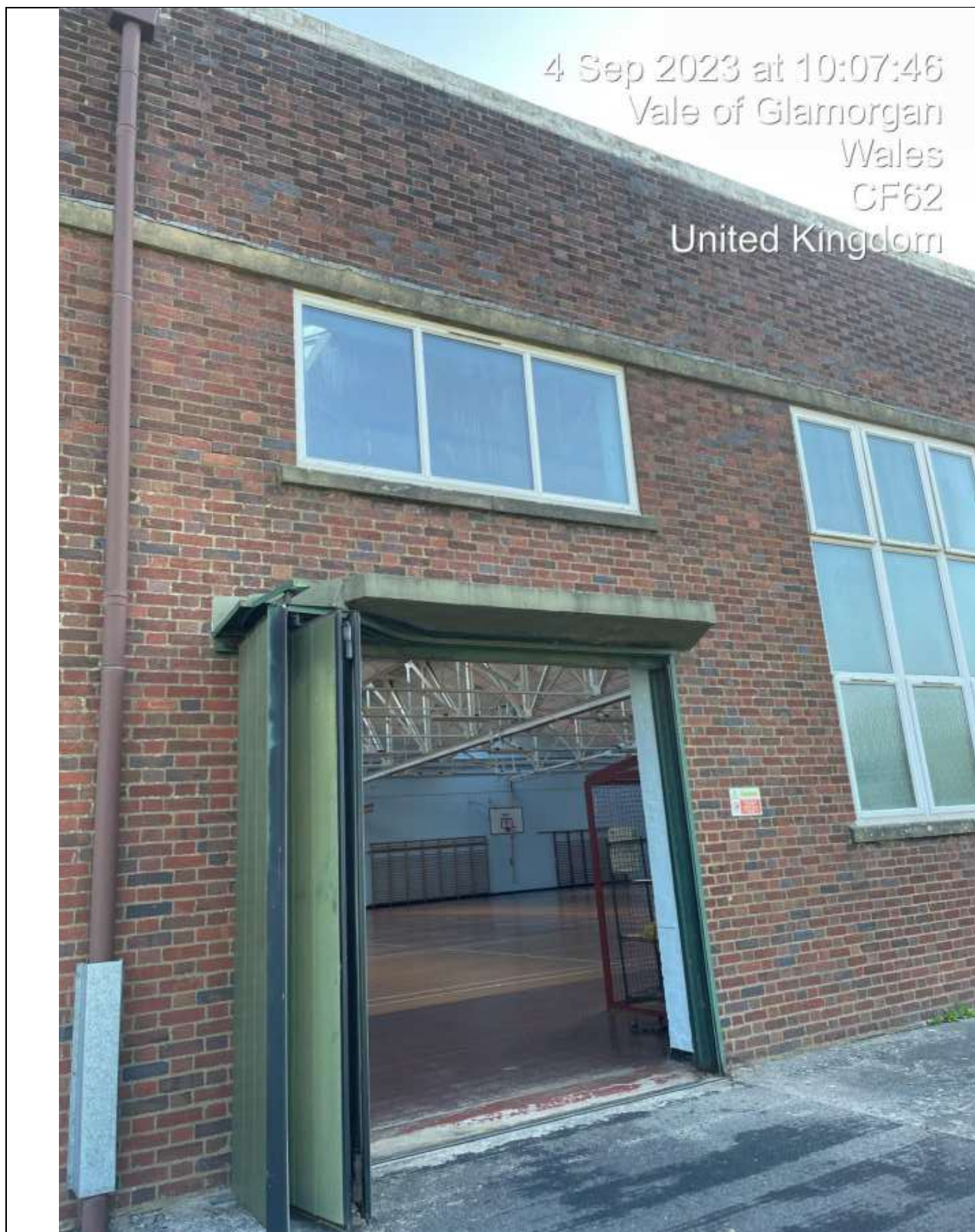
Western Elevation. Access & Egress Point.
