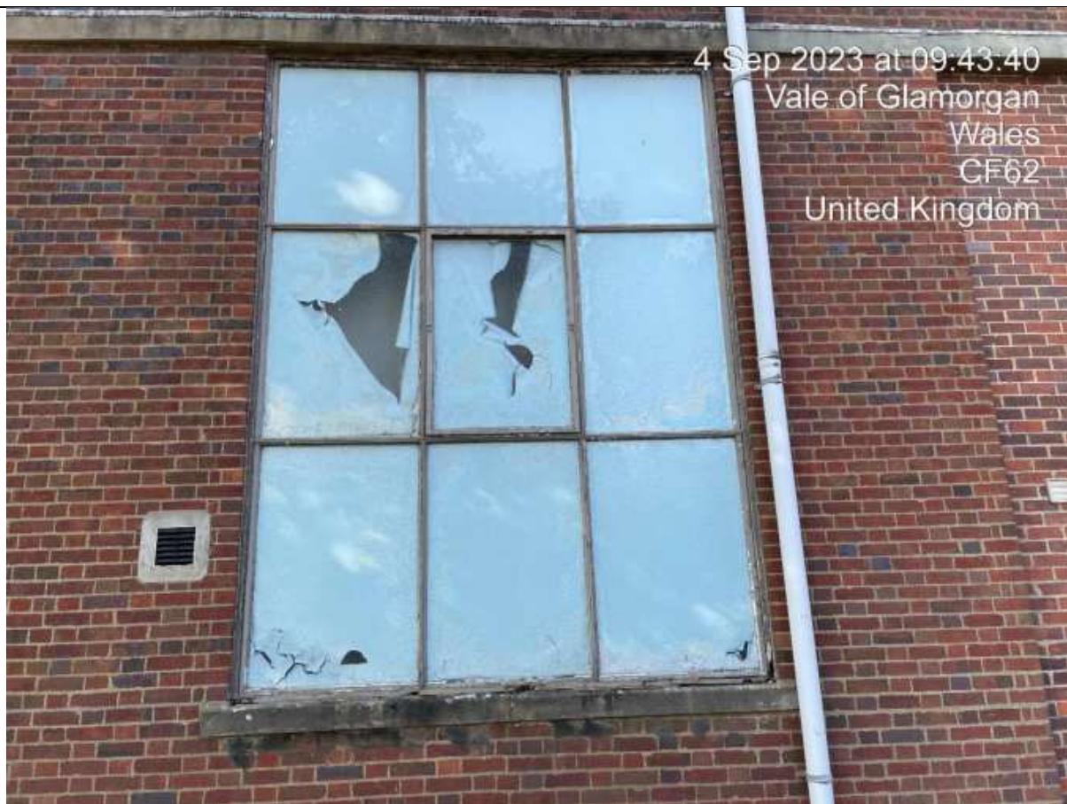
Eastern Elevation. Original Fenestration Covered Internally.
