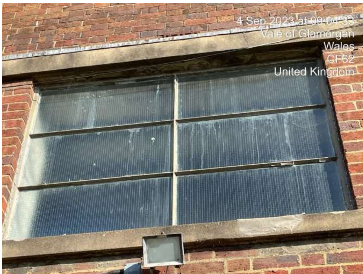
Southern Elevation. Original Fenestration but Non-Original Glazing.
