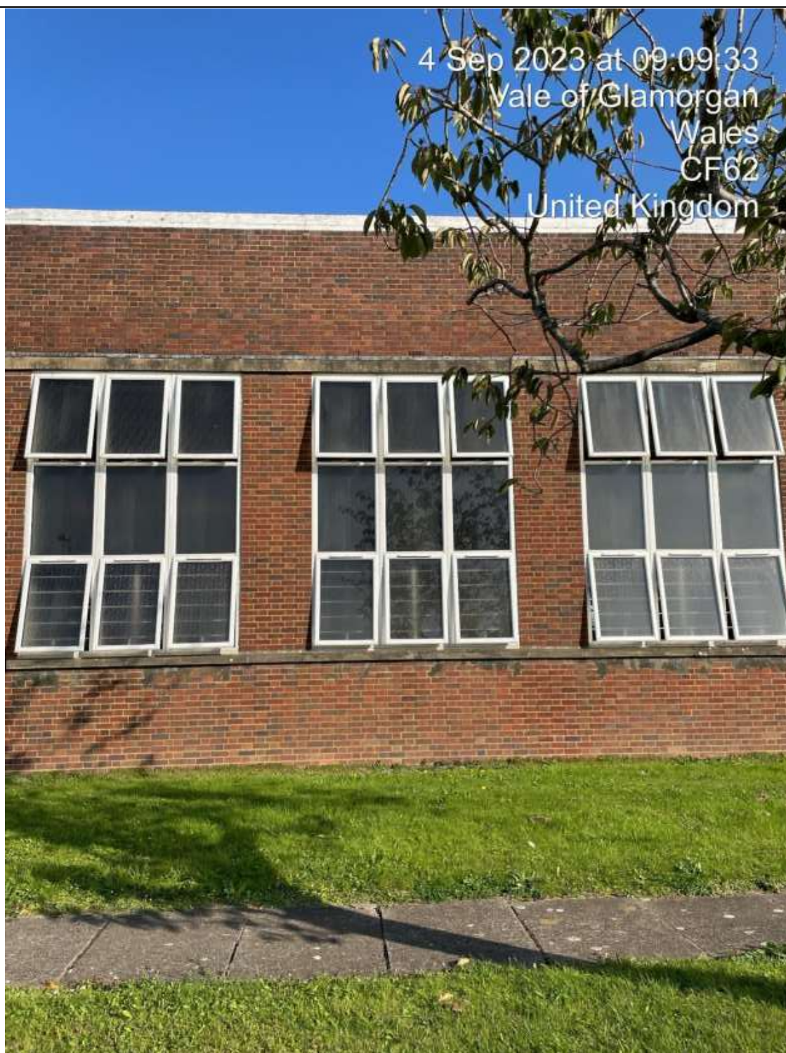
Southern Elevation. Replacement Fenestration.
