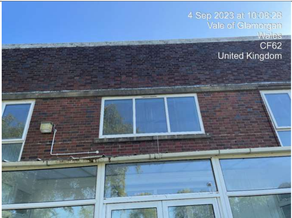
Western Elevation Replacement Fenestration.
