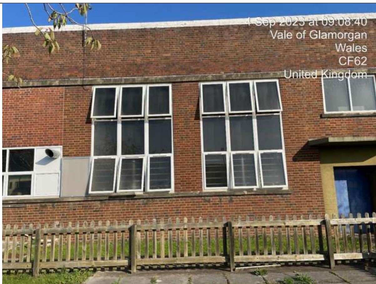
Southern Elevation. Note the Replacement Brickwork & Replacement Fenestration.
