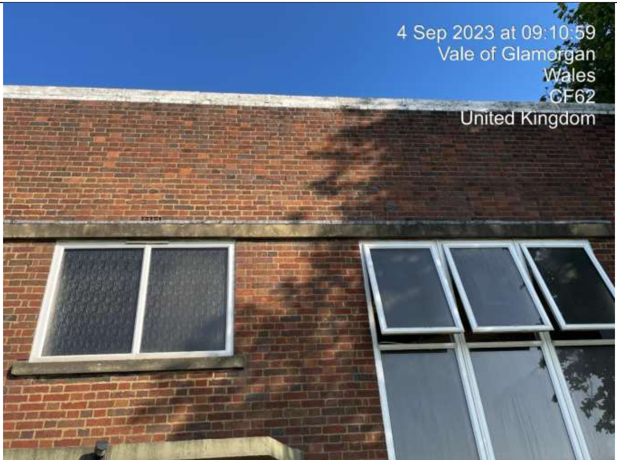
Southern Elevation. Replacement Fenestration.
