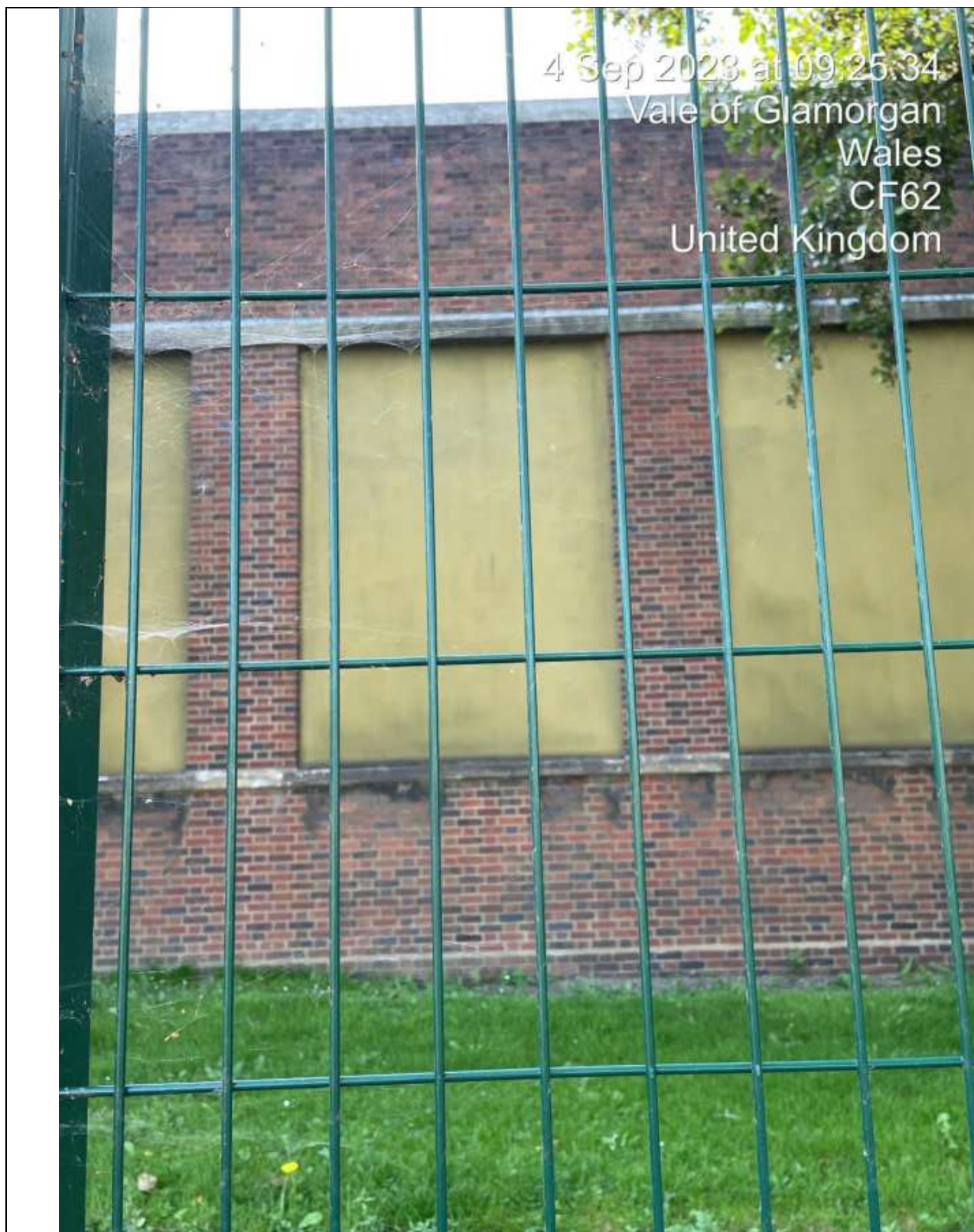
Northern Elevation. Blanked Off Fenestration.
