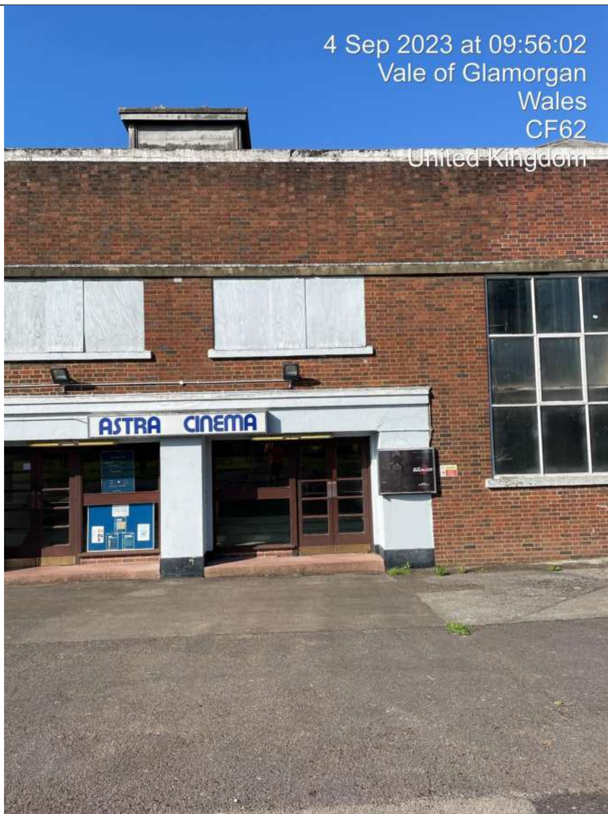
Eastern Elevation. Non-Compliant Access & Egress Points.
